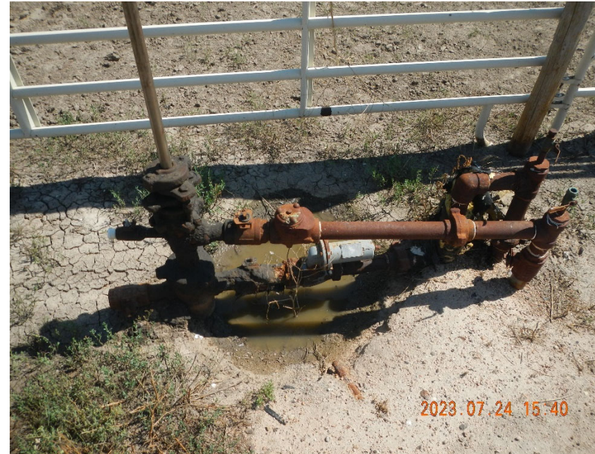
2. Wellhead. Note debris at wellhead and stained impacted soils around wellhead.
