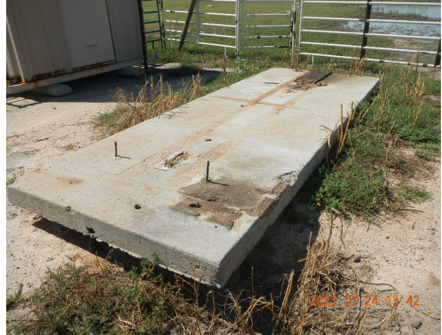
4. Concrete pad. Note staining and crusted lube oil on pad. Stained impacted soil around pad.
