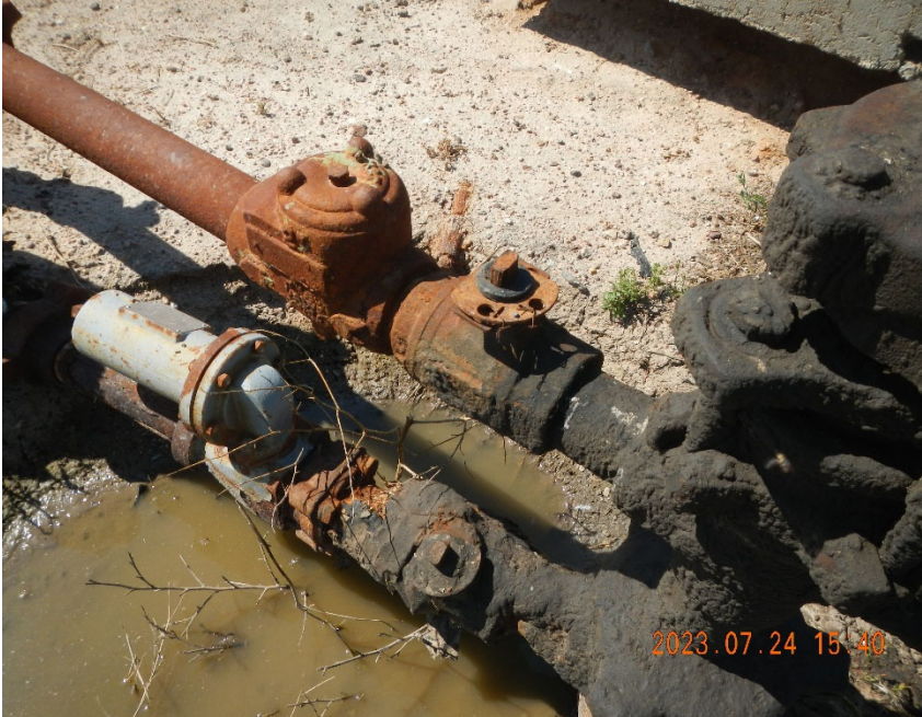
3. Closer view of Wellhead. Note stained soils and crusting on wellhead itself.
