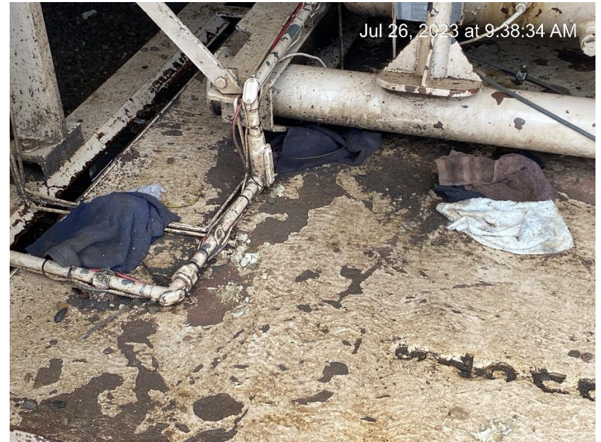
Debris and oil around compressor
