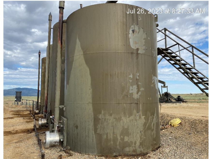
Oily waste covering tank and on the ground
