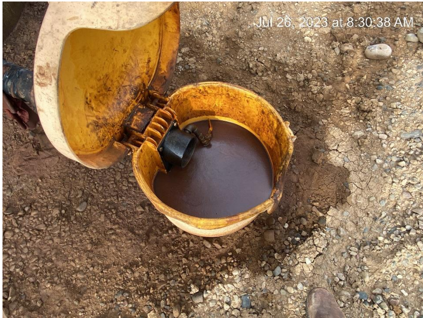
Open end loadline and full of oil
