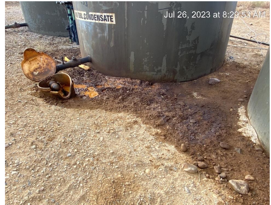
Debris, oily waste and stained soil
