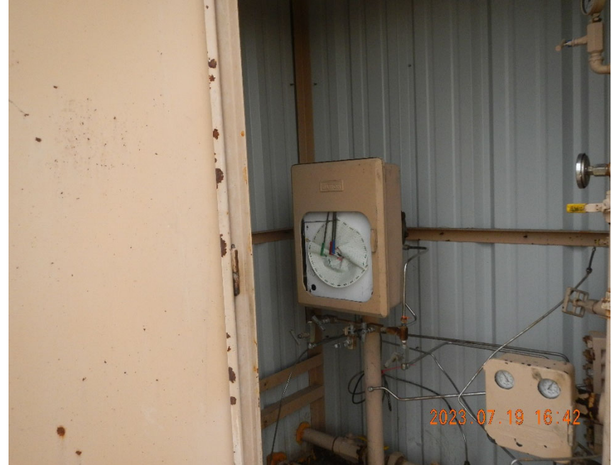
6. View of Gas Meter Run inside Meter Shed. Note there is no Meter Calibration/Test log attached to meter.
