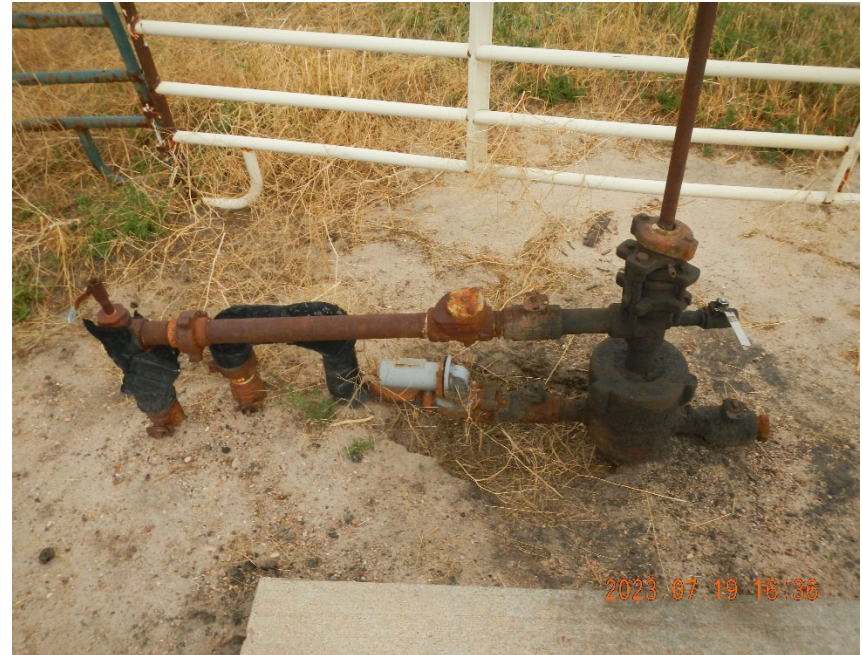
2. View of Wellhead. Note stained and impacted soils around wellhead.
