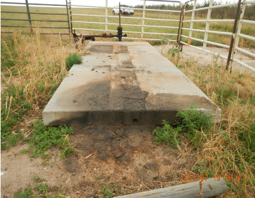
5. View of concrete pad from rear looking towards wellhead. Note staining on pad and ground around pad.
