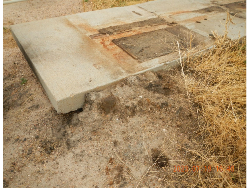
4. Concrete pad (Pump Jack). Note staining on pad and ground around pad.
