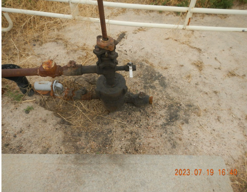
3. Closer view of stained and impacted soil around wellhead.
