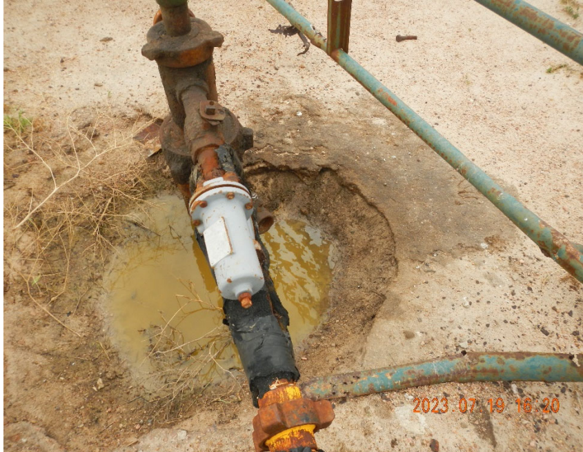
3. Close up view of stained soil and oily fluid around bottom of wellhead.
