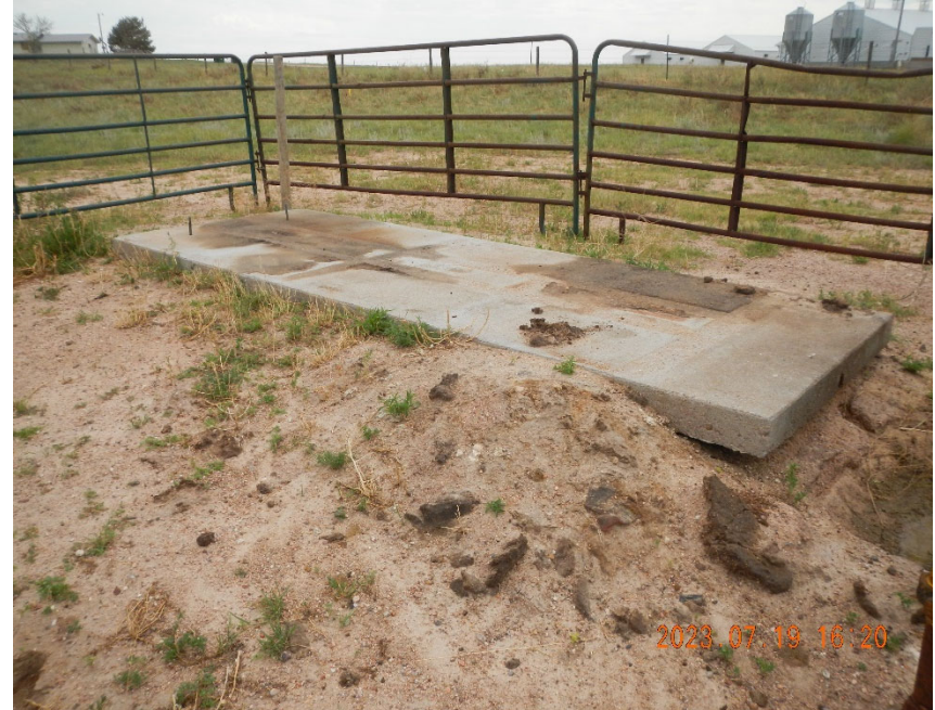
4. Concrete pad (Pump Jack). Note stained and impacted soil around edge of cement pad and encrusted lube oil patches on surface of concrete pad.
