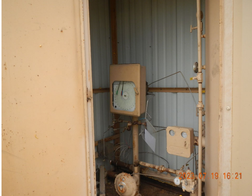
5. Gas Meter Run inside Meter Shed.
