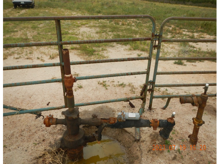
2. View of wellhead. Note staining on soil and fluid around base of wellhead.
