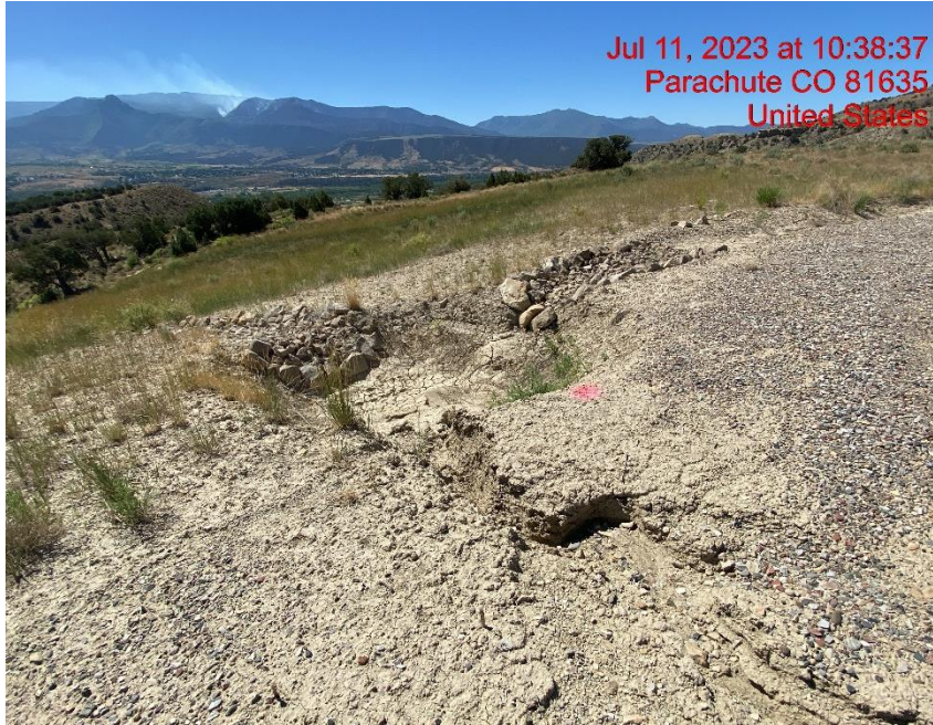
Inadequate Erosion Control of Location Surface – Photo #05184
