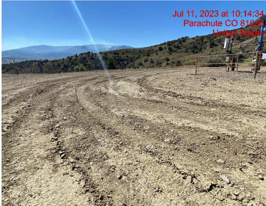
Location Lacks Stabilization – Photo #05153
