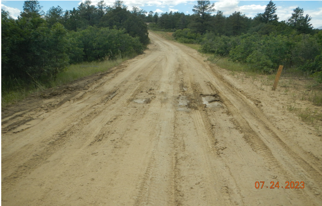
Photo 2. Facing northwest along the main road. Stormwater is pooling in this area causing vehicle rutting and widening of the road.
