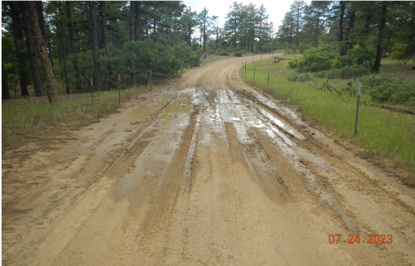
Photo 3. Facing northwest along the main road. Stormwater is pooling in this area causing vehicle rutting and erosion.
