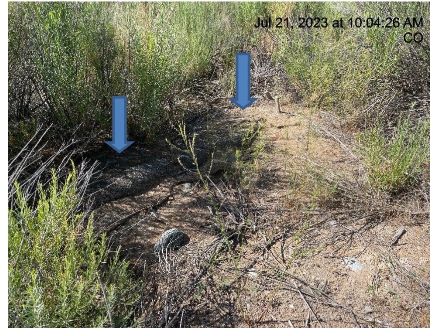
Photo # 3589 Wattles need maintenance (S/SW area of location)
