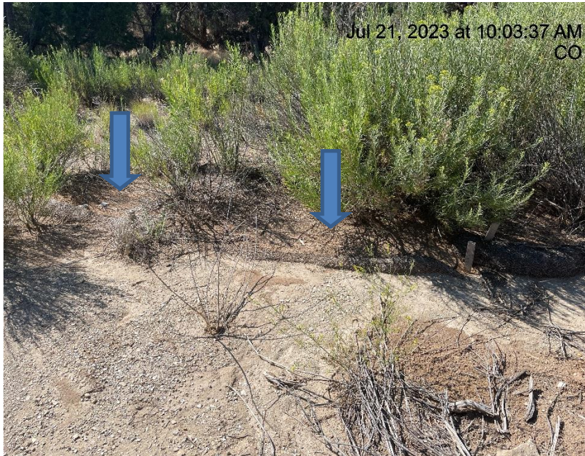
Photo # 3586 Wattles need maintenance (S/SW area of location)
