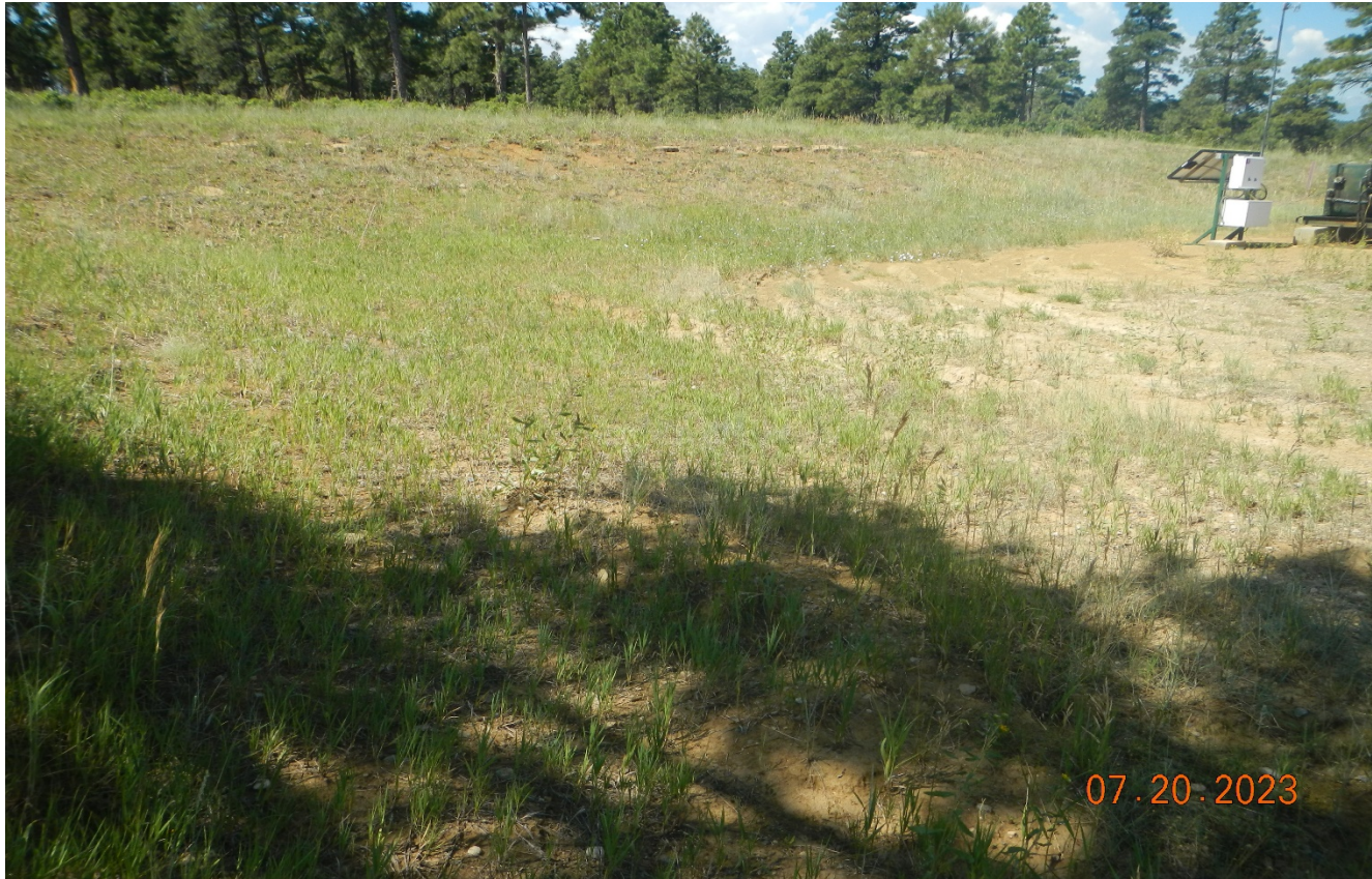
Photo 3. Facing toward the cut slope which is stabilized with vegetation.
