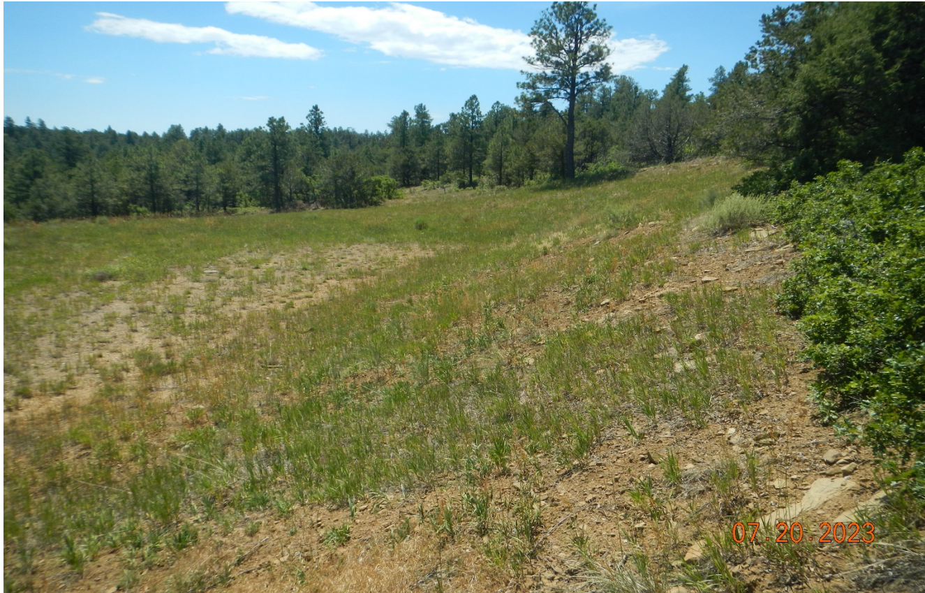
Photo 2. Facing along the cut slope of the location which is stabilized with perennial vegetation.
