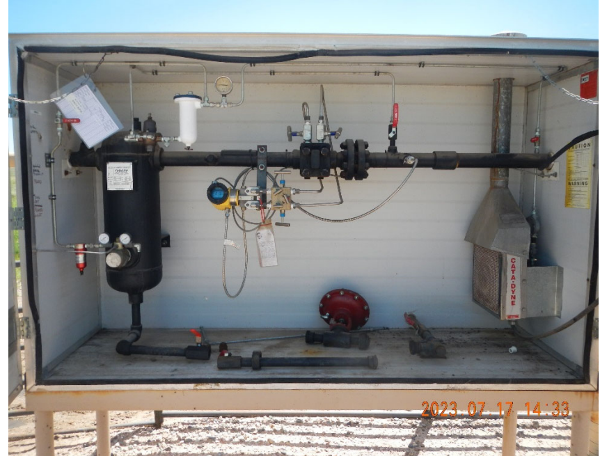
6. View of Digital Gas Meter Run inside equipment cabinet.
