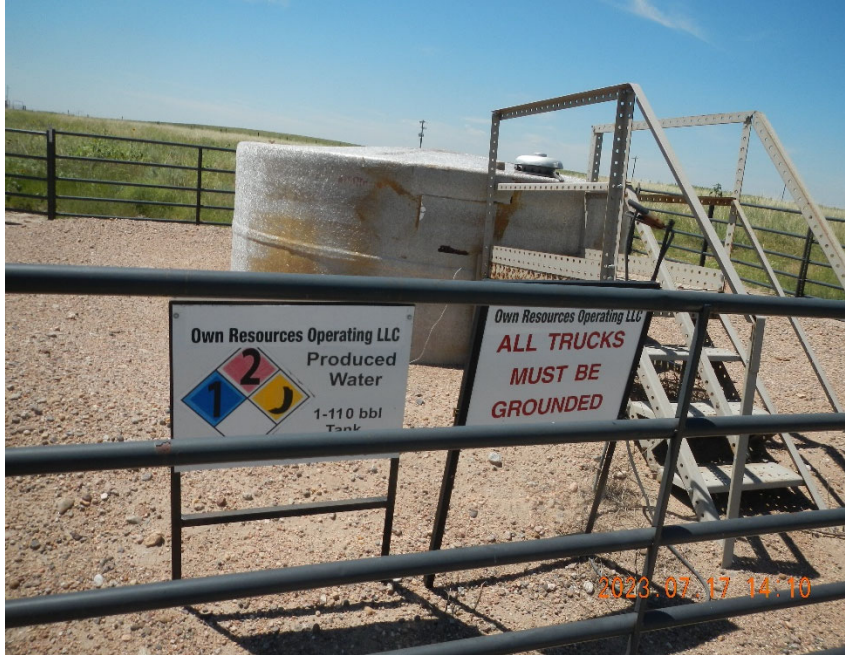
5. Signage inside fencing at front of produced water tank.
