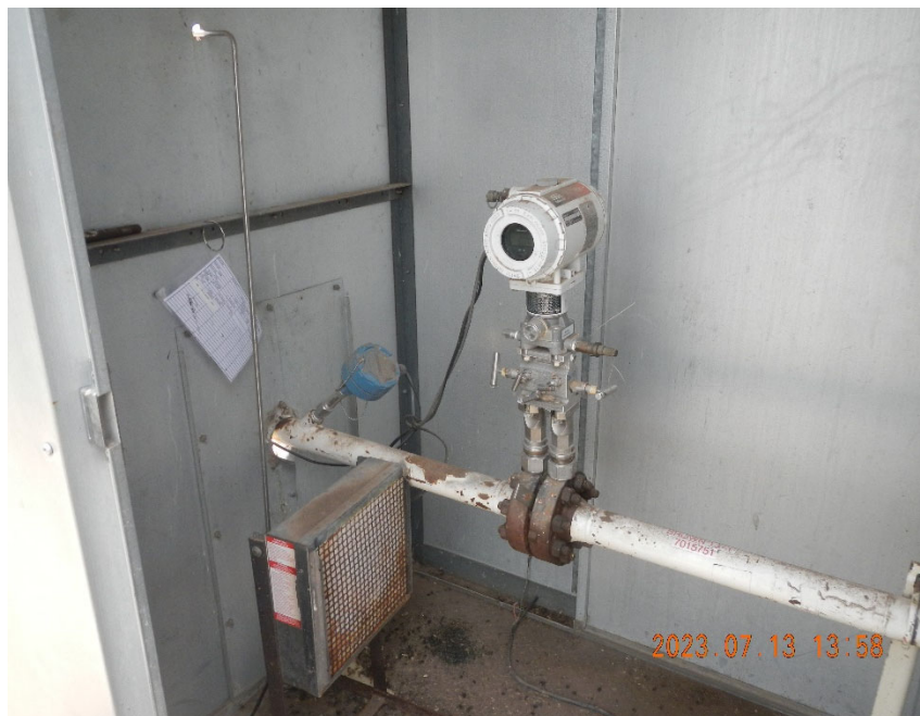
5. Digital Gas Meter Run.
