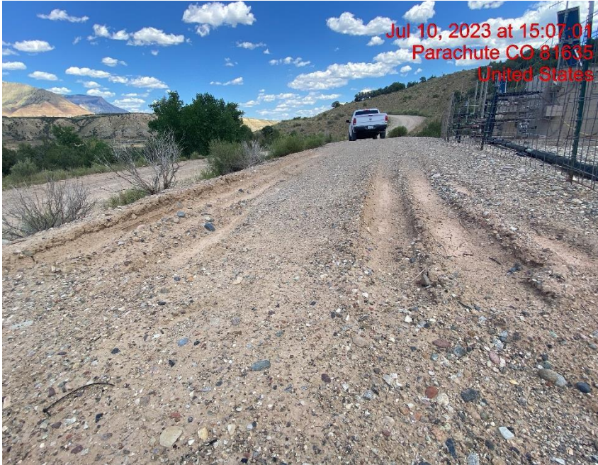
Lack of Stabilization – Photo #05123
