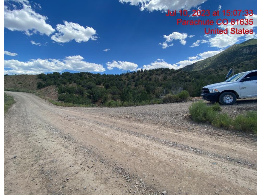
Insufficient Vehicle Tracking BMPs at Location Entrance/Exit – Photo #05124
