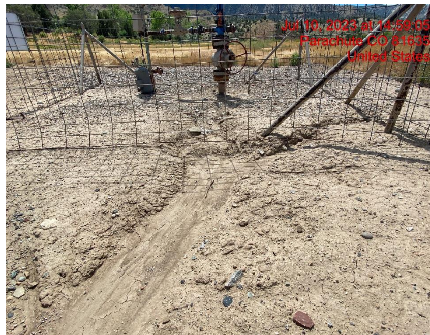
Rill Erosion Causing Run-On to Location – Photo #05113
