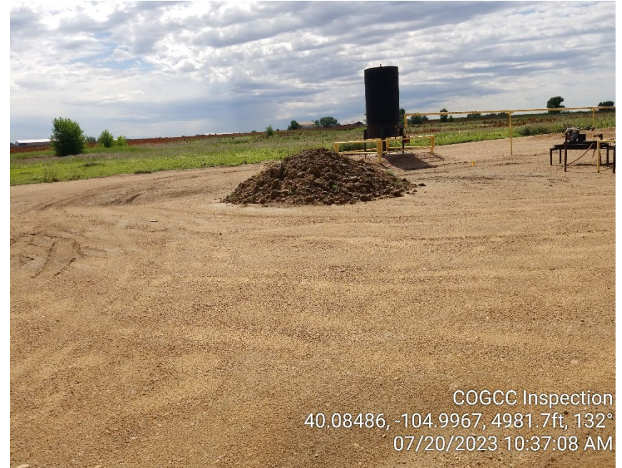
Photo 4 – Unlined soils pile with no BMPs.
