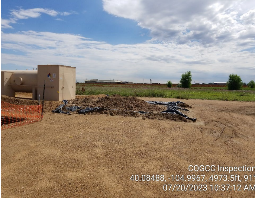
Photo 5 – Soils pile on liner.
