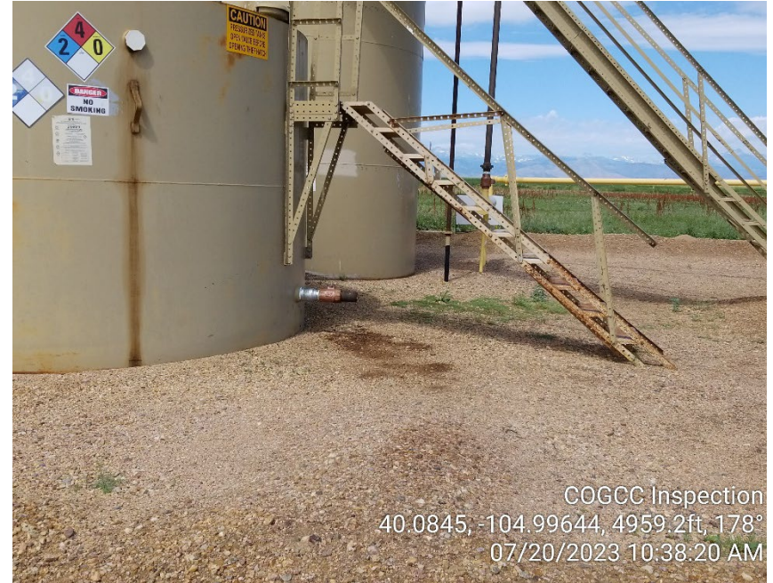
Photo 6 – Stained soil noted in inspection doc no 691201675.
