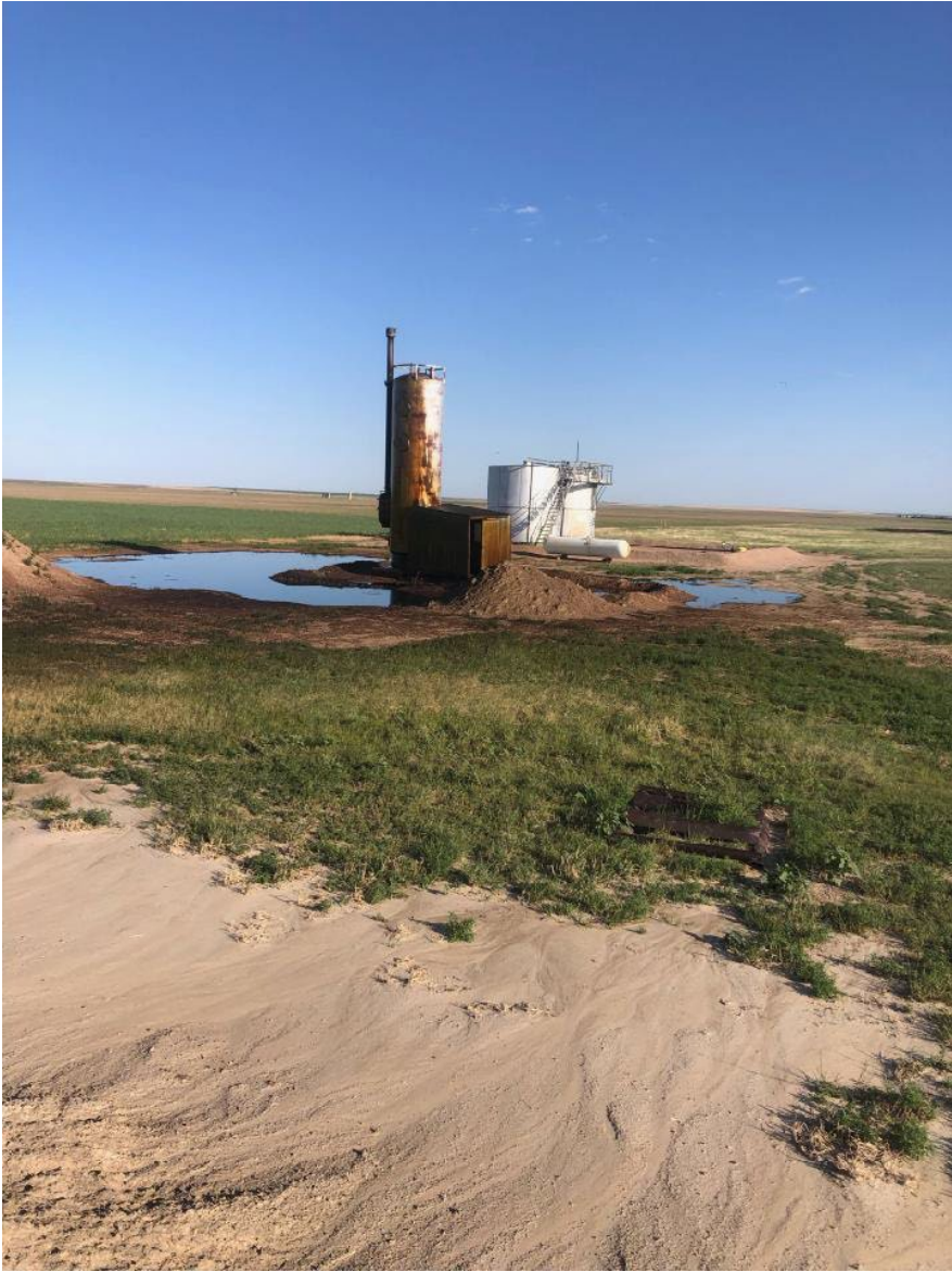
Photo 1 Initial Spill Photo
