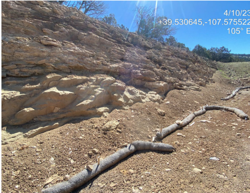
Waddles failing from previous inspection
