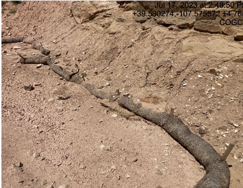
Waddles failing from recent inspection
