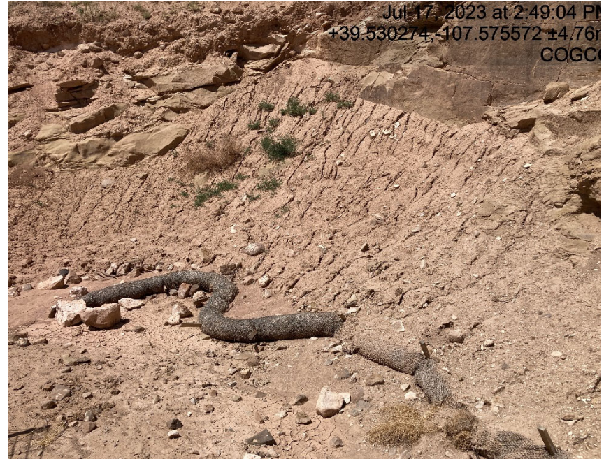
Waddles failing from recent inspection and erosion
