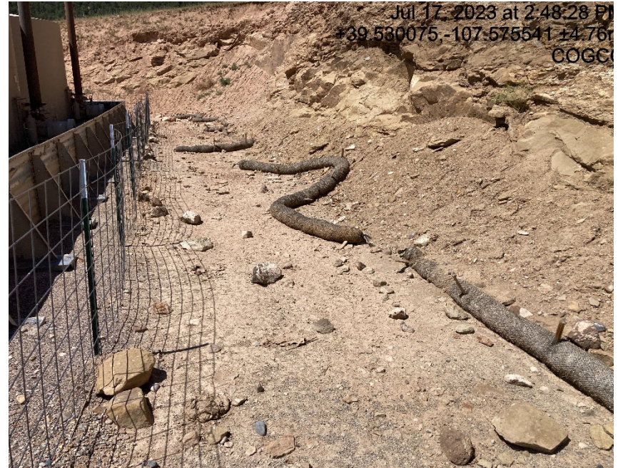
Waddles failing from recent inspection
