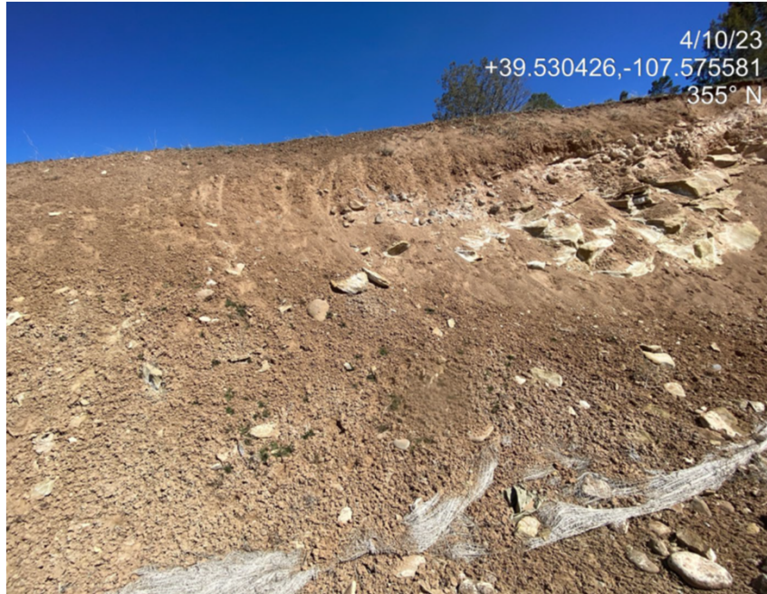
Erosion blanket from previous inspection and lack of stabilization.
