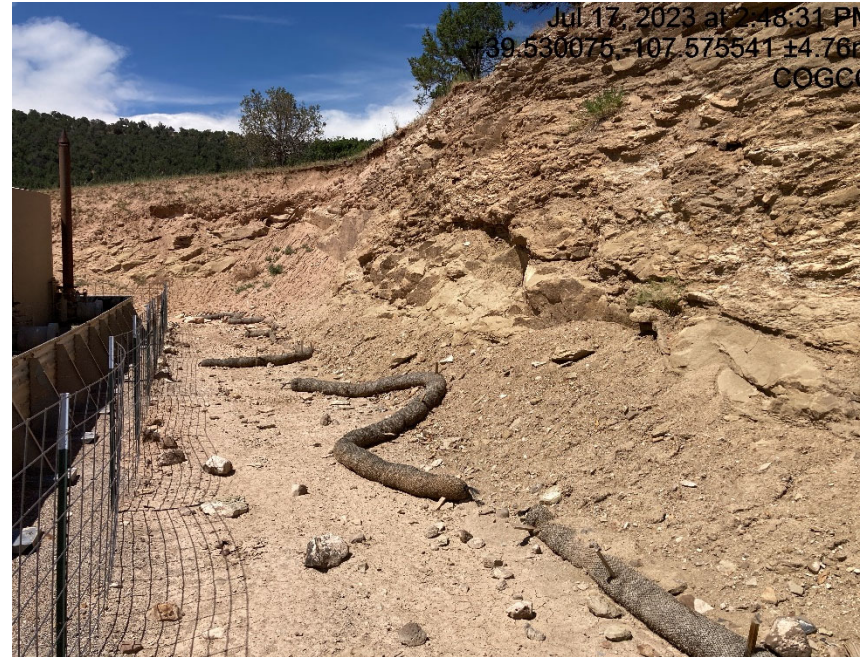
Waddles failing from recent inspection and lack of stabilization/ erosion
