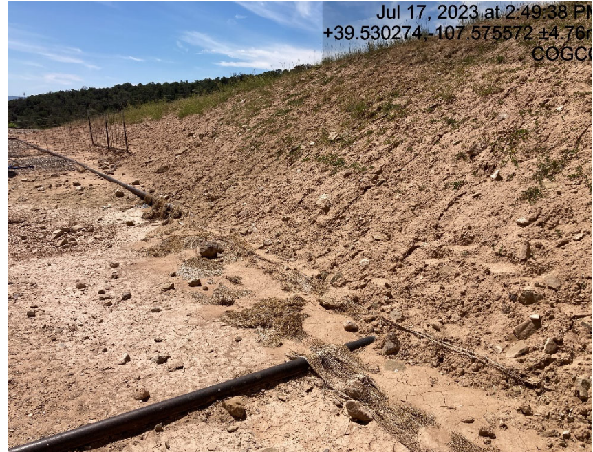
Erosion blanket from recent inspection and lack of stabilization.
