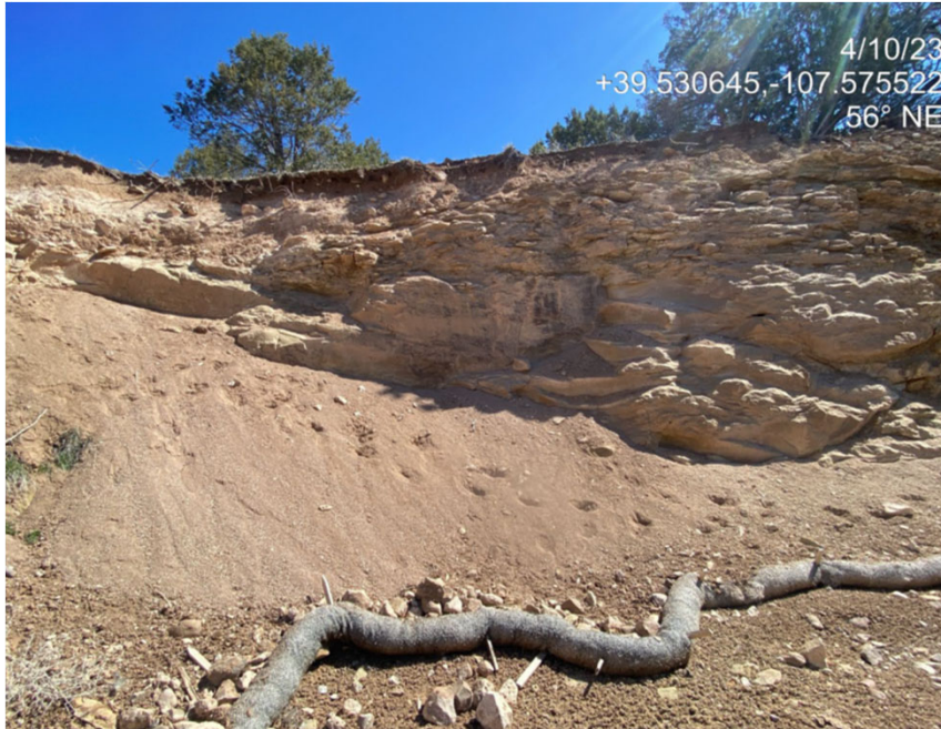
Waddles failing from previous inspection and lack of stabilization/ erosion
