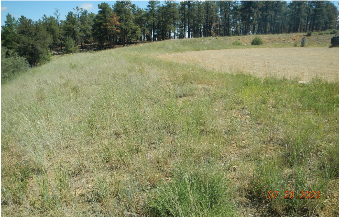
Photo 3. Facing northeast along the fill slope which is stabilized with perennial vegetation.
