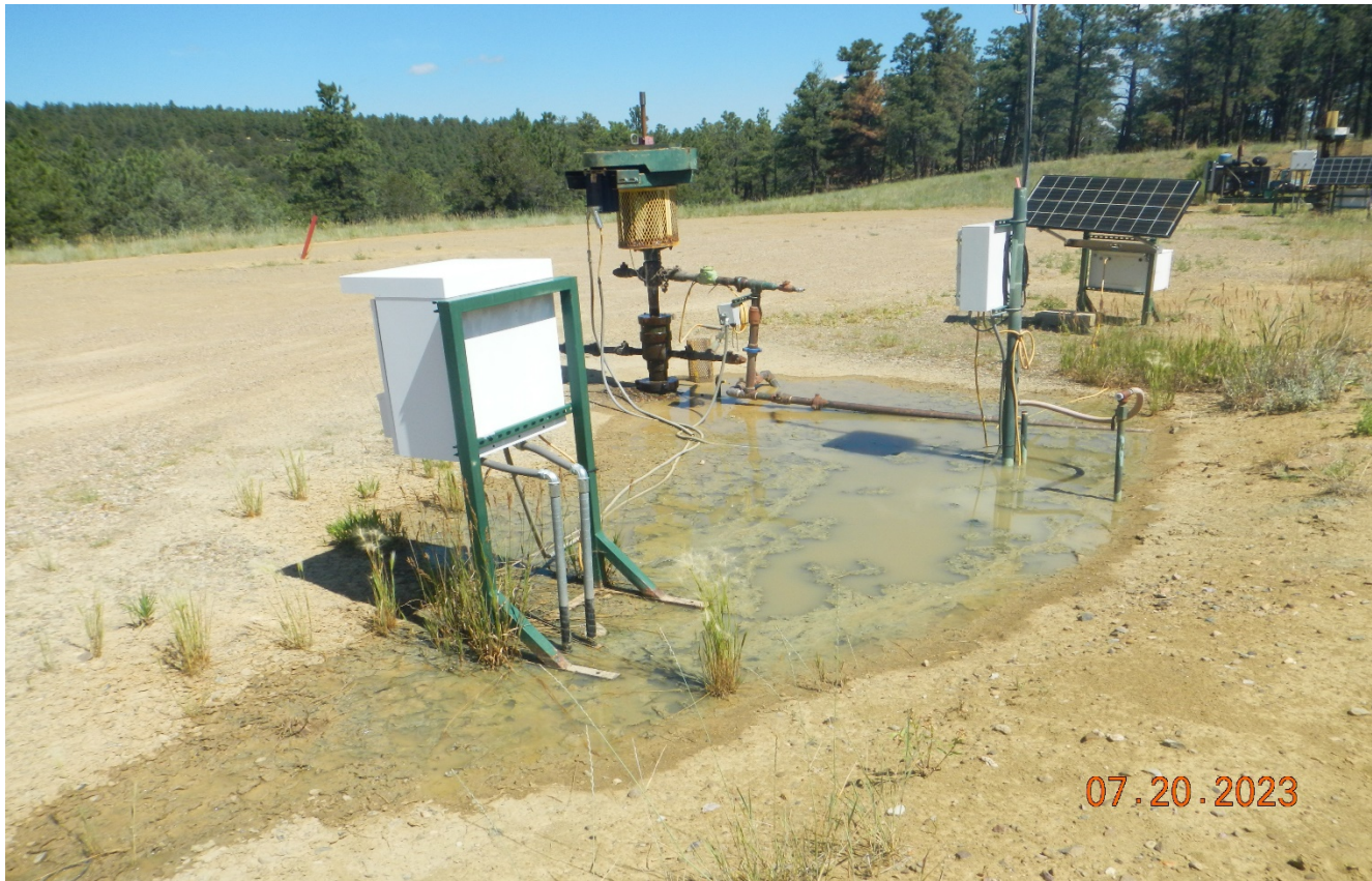
Photo 2. There is a dripping water leak at the wellhead that needs to be repaired.
