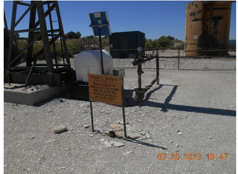
Injection wellhead
