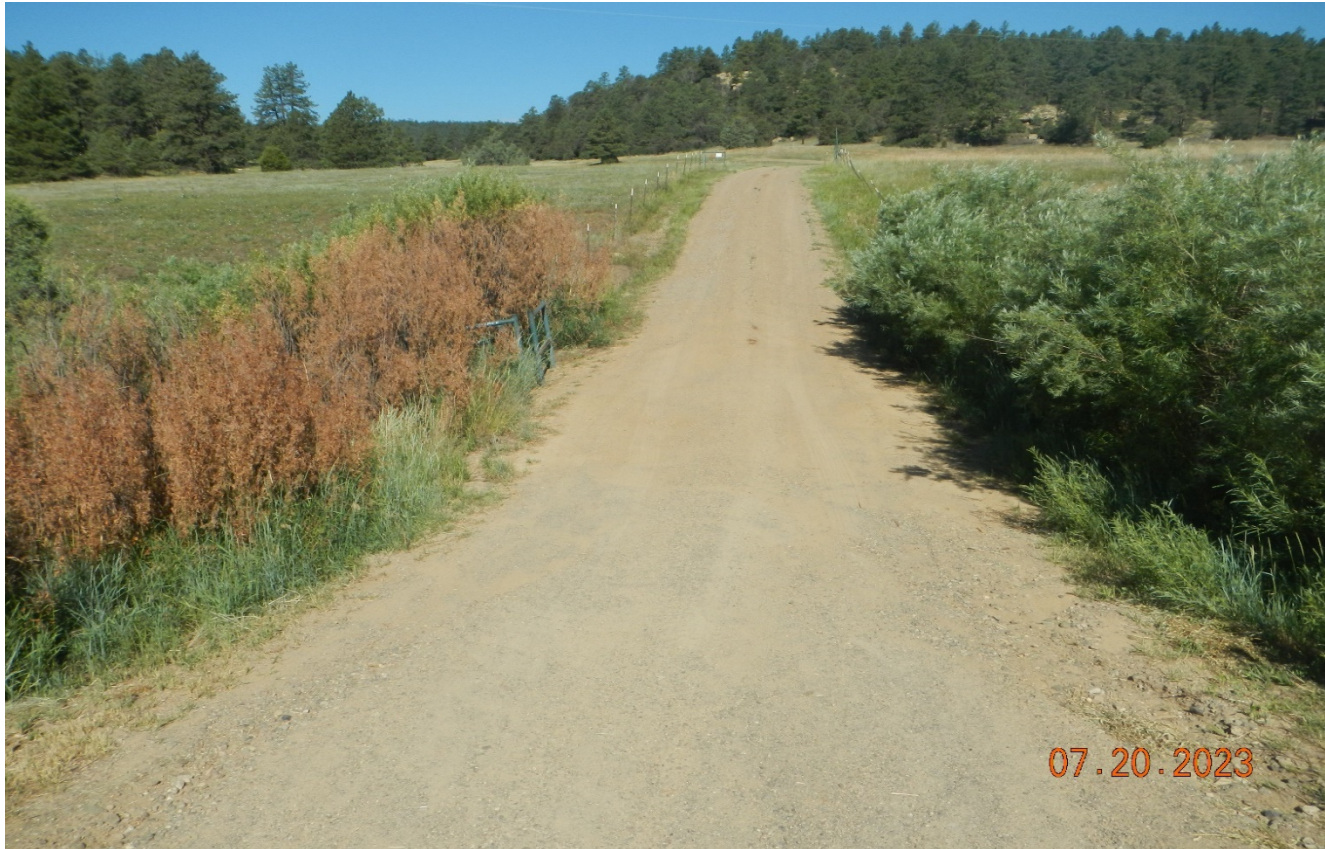
Photo 1. Facing west at the beginning of the access road. The willows along the road side have died from what appears to be incorrectly applied herbicide treatment.
