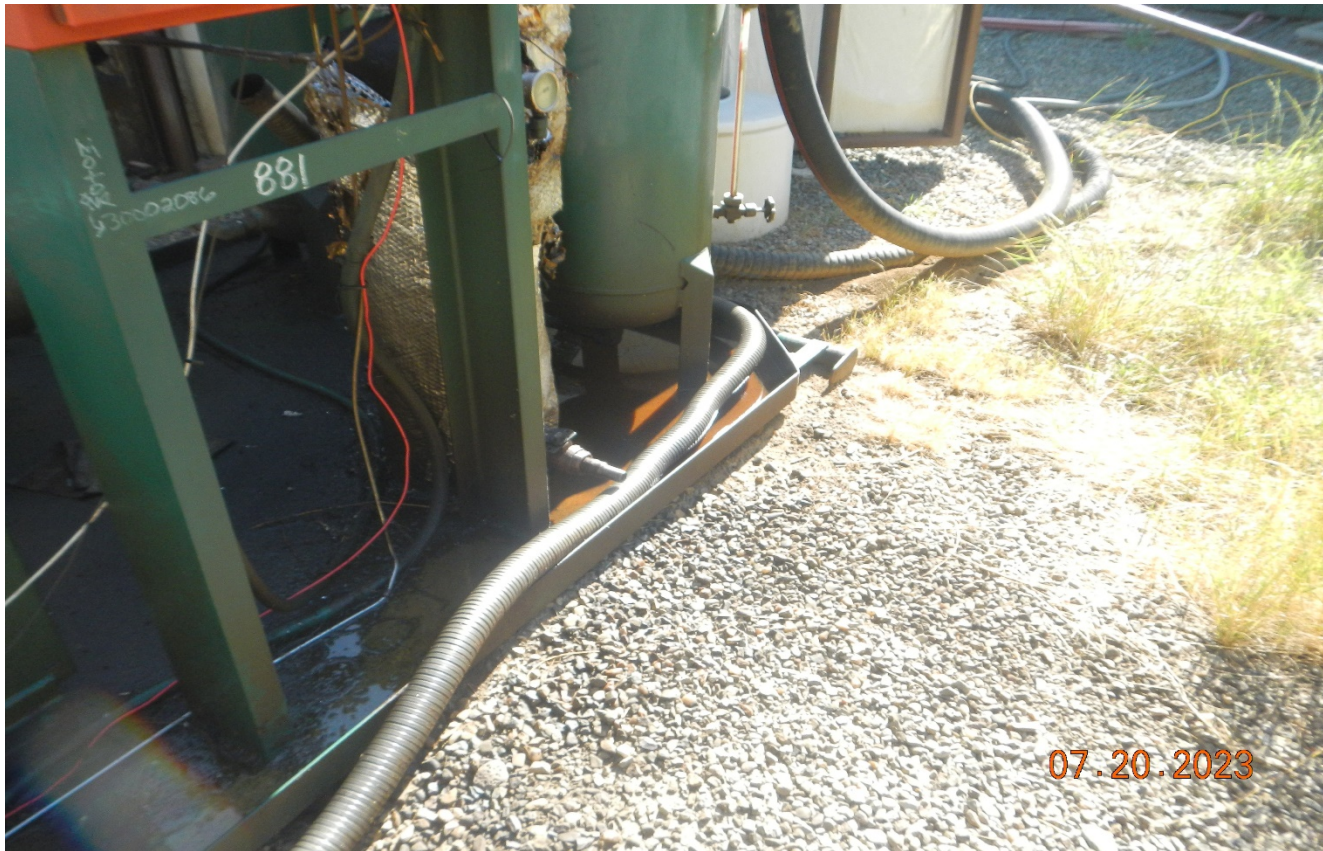
Photo 10. There is oily fluid in the engine skid that needs to be cleaned up.
