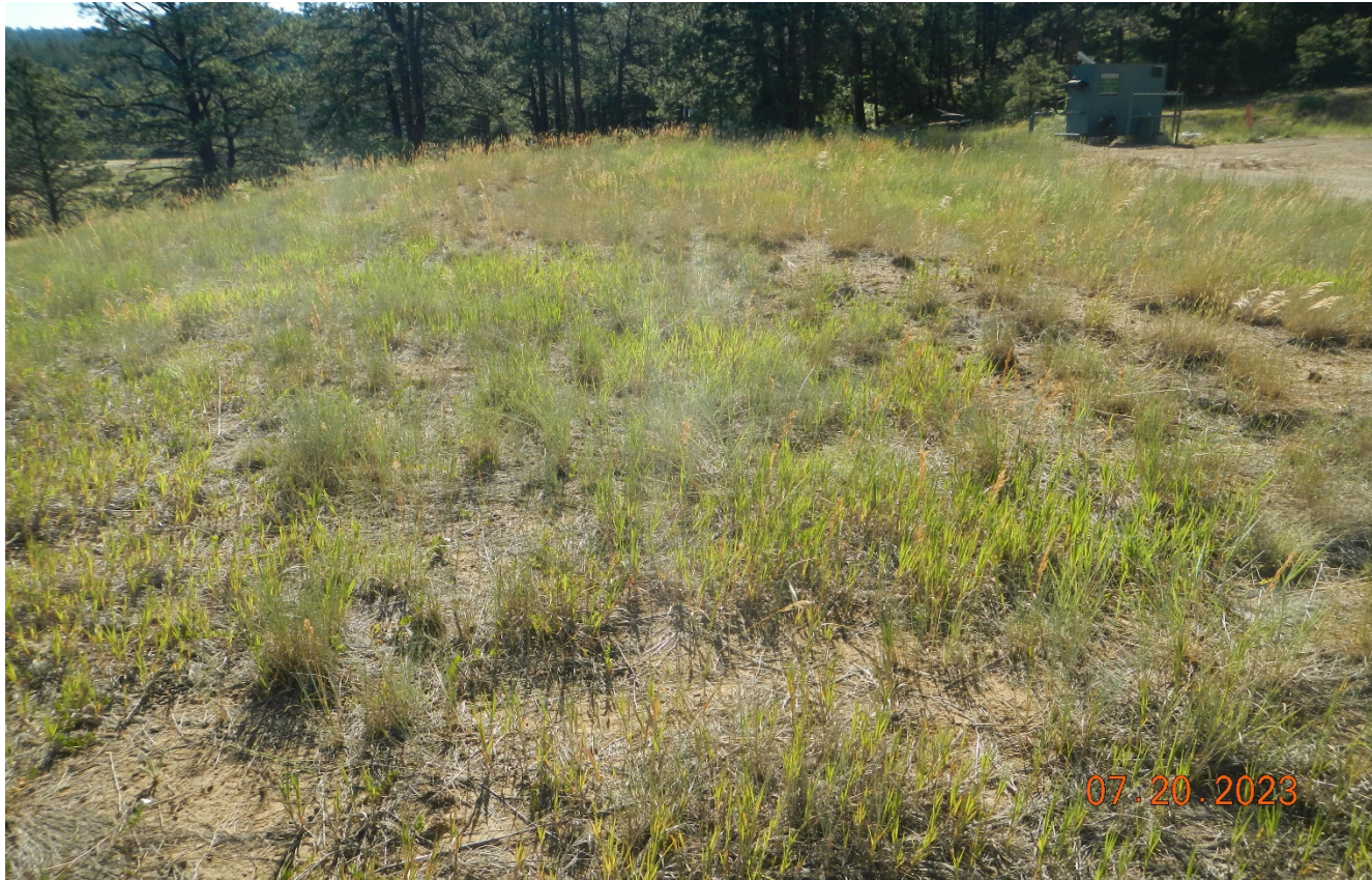
Photo 6. Facing southeast along the fill slope which is stabilized with perennial vegetation.
