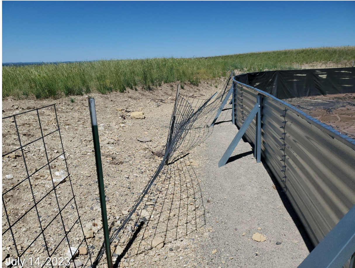
Photo 1: Fence at battery in disrepair.
