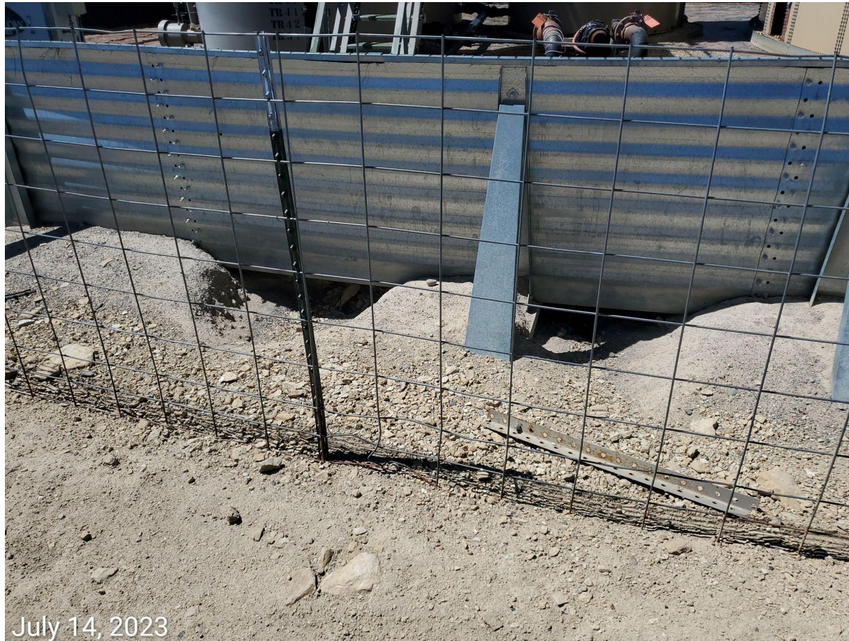
Photo 2: Evidence of wildlife burrowing under containment BMP
