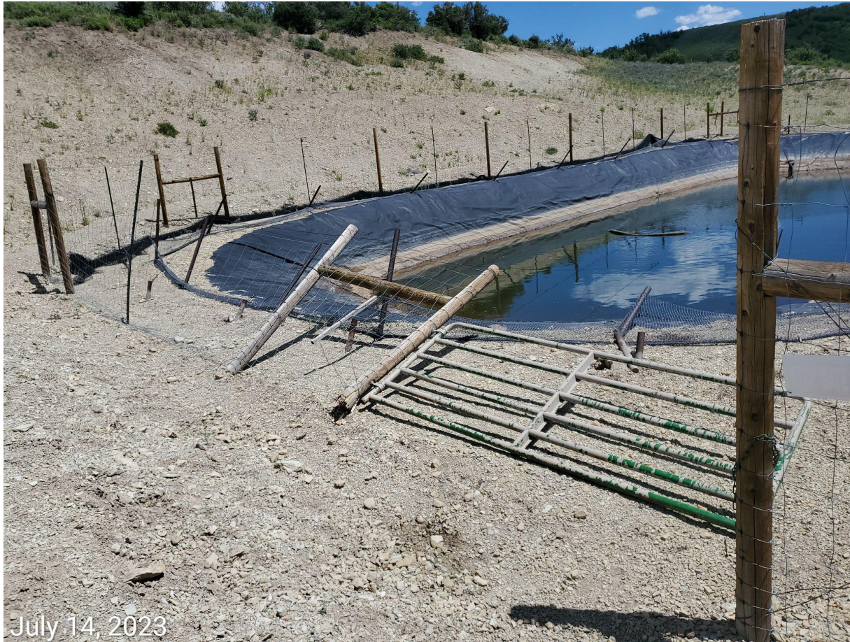
Photo 3: Fence at pit in disrepair.
