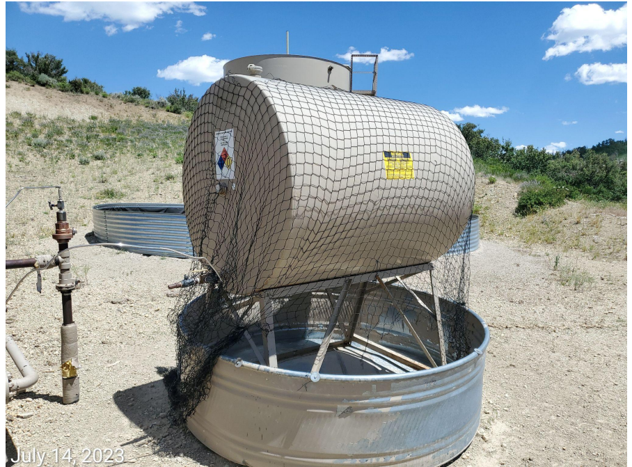
Photo 6: BMPs to prevent wildlife remain missing, or in disrepair at containment BMPs
