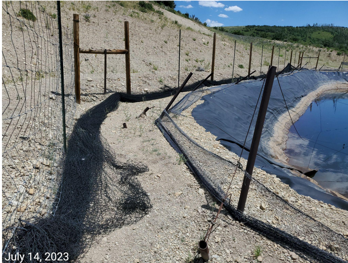
Photo 5: Netting at pit stored on edge of pit.
