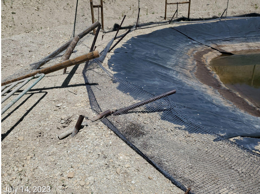
Photo 4: Fence/netting at pit in disrepair.
