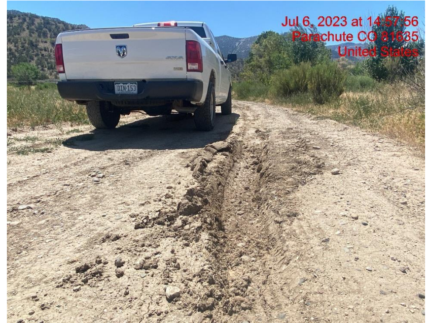
Lack of Stabilization – Photo #05034
