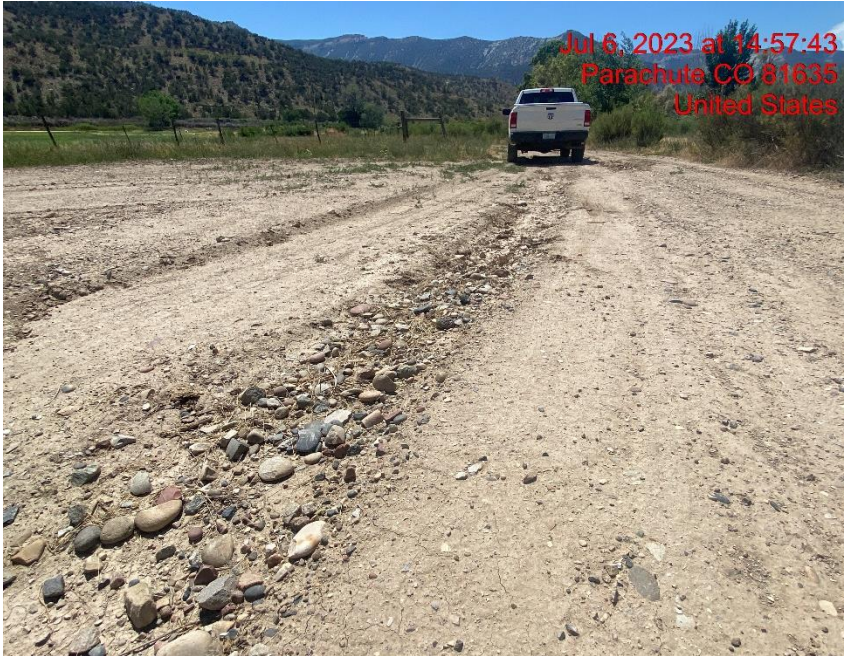
Lack of Stabilization – Photo #05033
