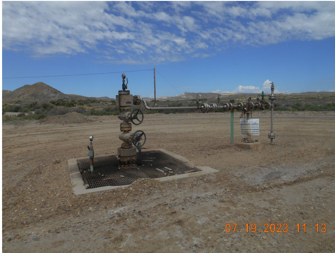
Injection wellhead
