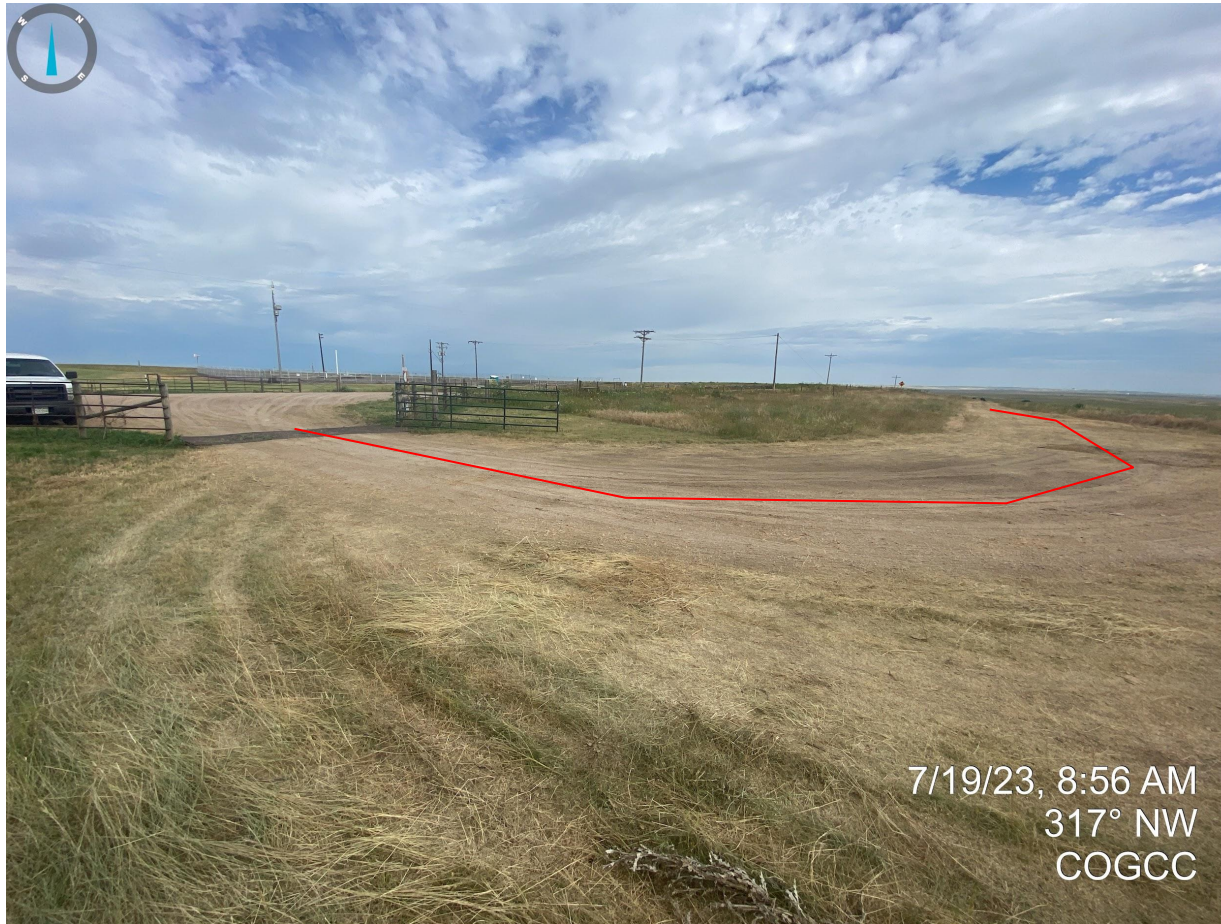
Photo 2. Portions of land experiencing vehicle traffic (red line) with no evidence of topsoil salvage having occurred. This entrance is approximately 1000' south of the current location entrance. Topsoil will need to be salvaged from this access point pictured if it's going to be used in future oil and gas operations, or, the disturbed areas will need to be reclaimed in accordance with 1000 series Rules.
