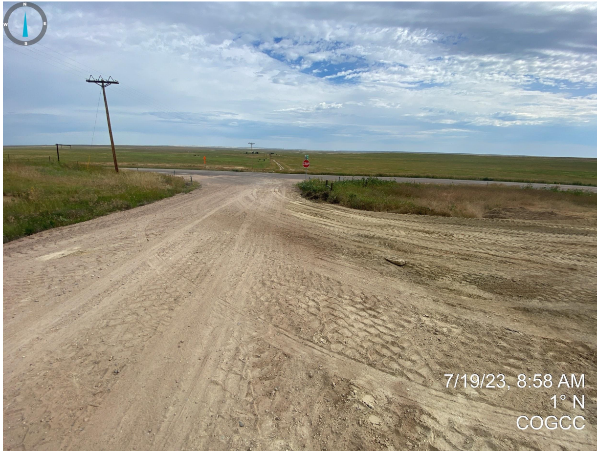
Photo 5. Facing north from the location's current access point. No BMPs observed to prevent vehicle track out. The location signage should be installed at the location's access road point and the intersection of an adjacent road.
