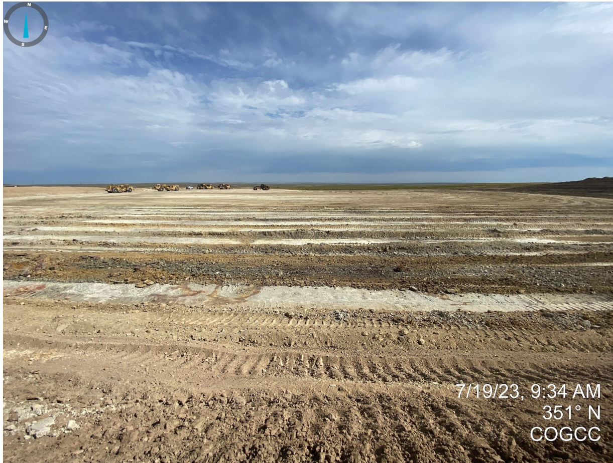
Photo 14. Overview of drilling pad area under construction.
