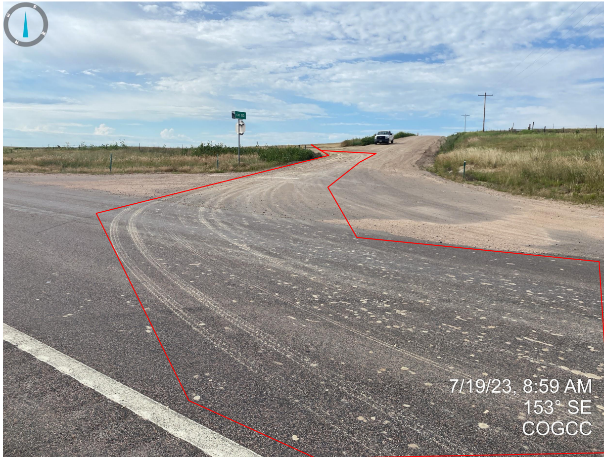
Photo 7. Facing southeast, see comments in Photo 6.
