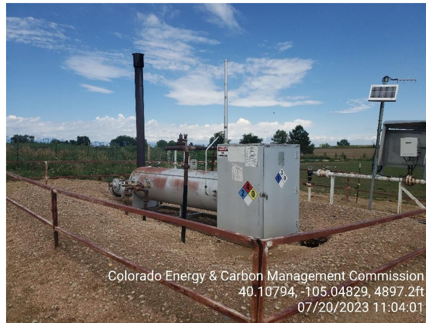
Photo 14 Horizontal heated separator.
