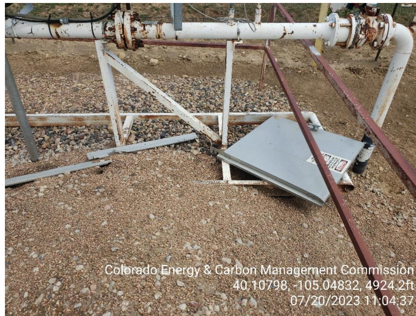
Photo 16 Gas Meter Run door and frame on the ground/trash.
