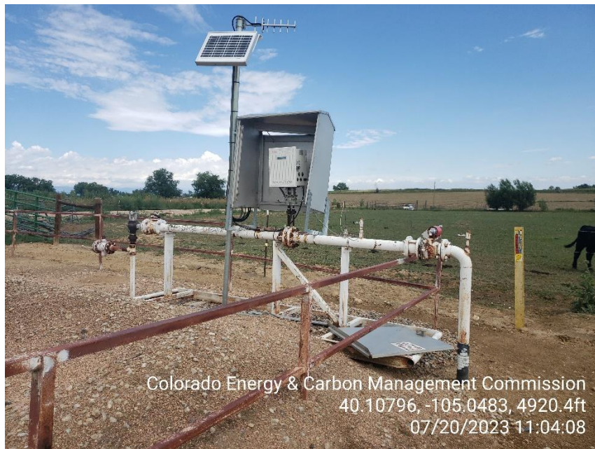
Photo 15 Gas Meter Run.
