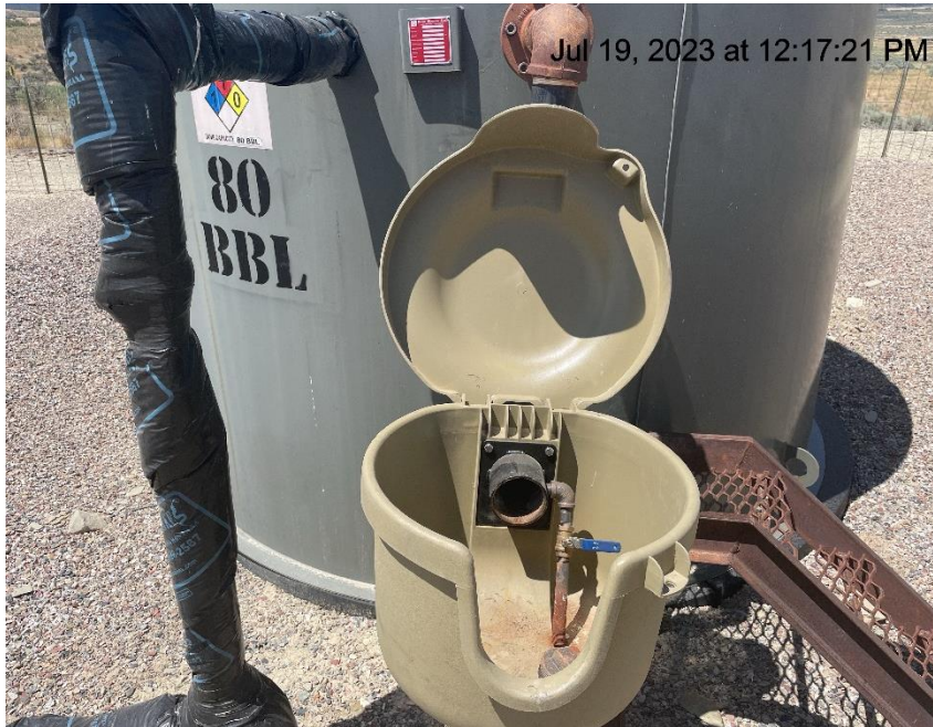
Photo # 3389 Open ended load line
