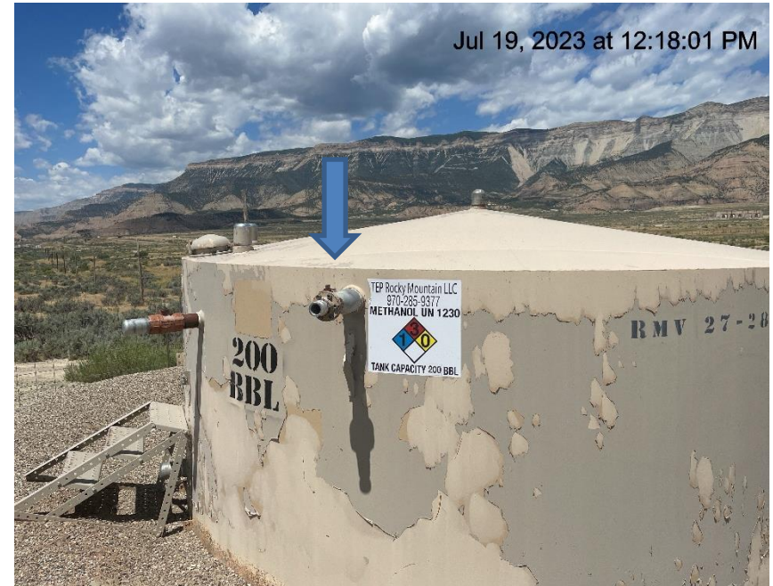
Photo # 3390 Open ended load line
