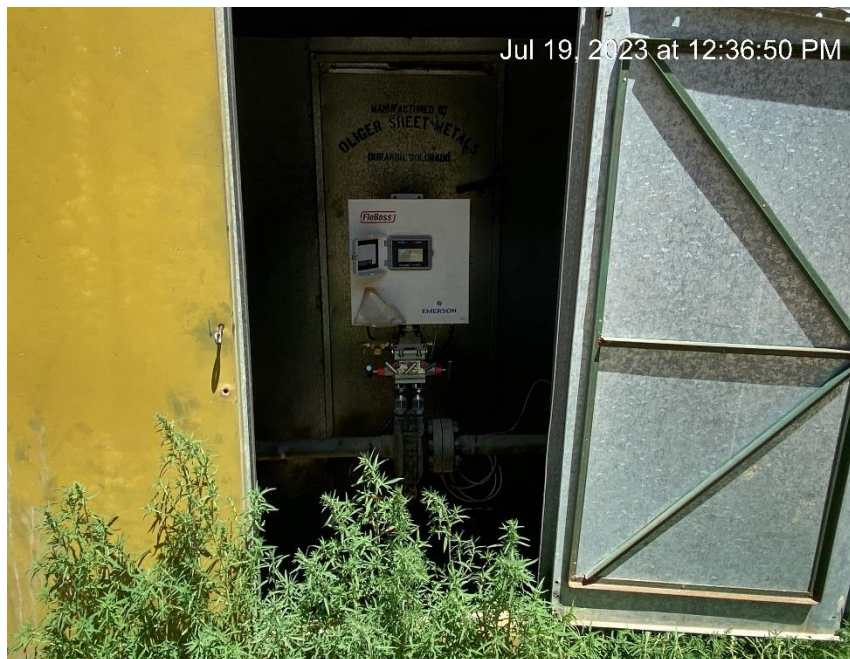
Gas meter calibration card not visibly displayed
