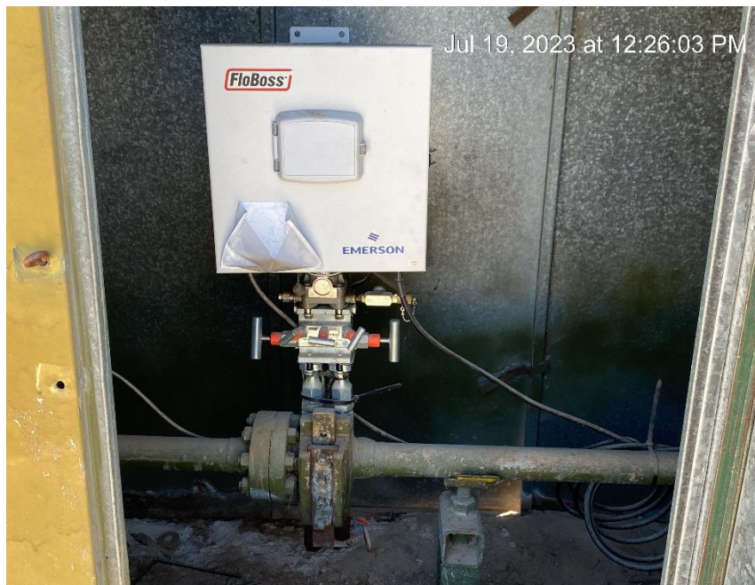
No visible display of gas meter calibration
