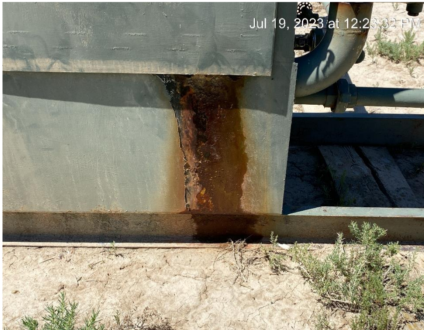
Separator leak
