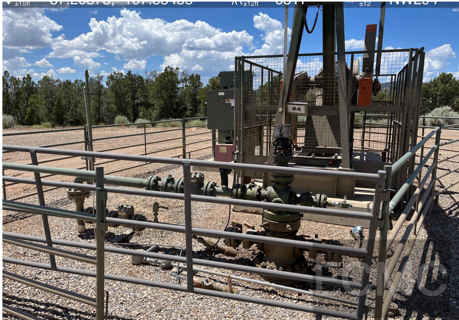
Photo #4. View of the #4 wellhead assembly.
