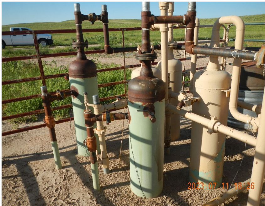
5. Gas Dryer Vessel at remoter Gas Meter Run.
