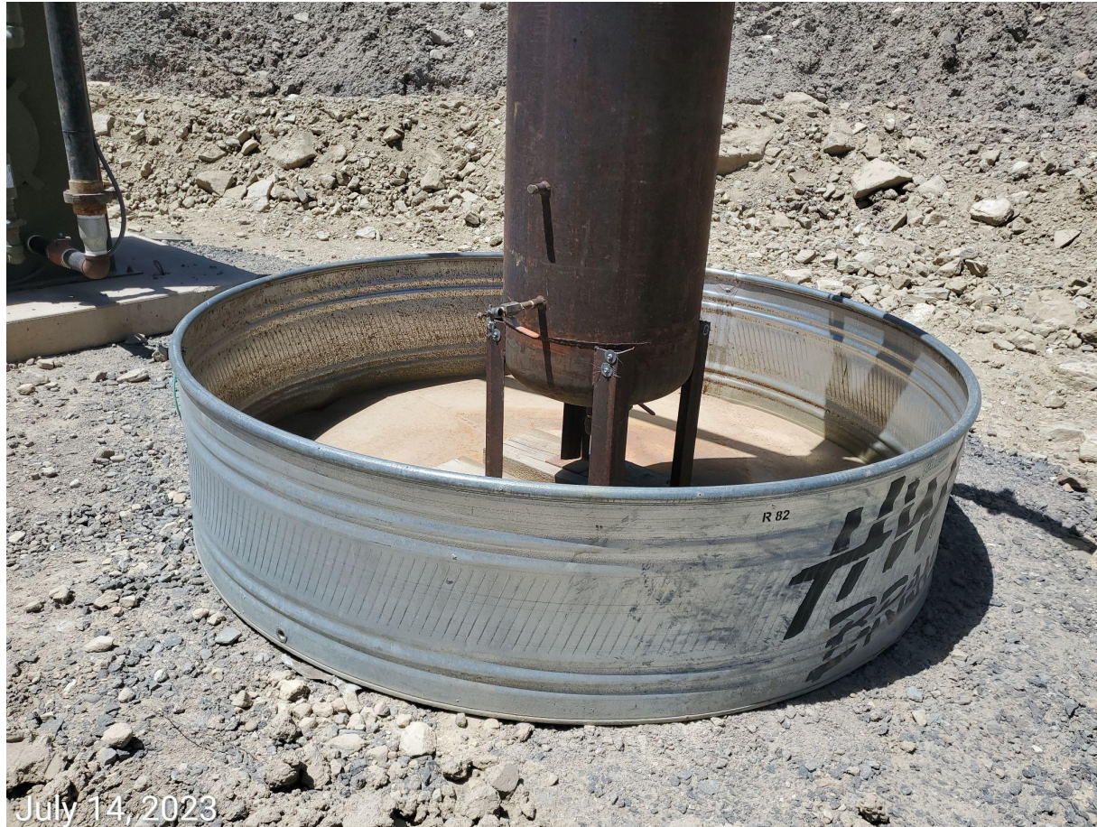
Photo 6: BMPs to prevent wildlife access missing from containment BMP.
