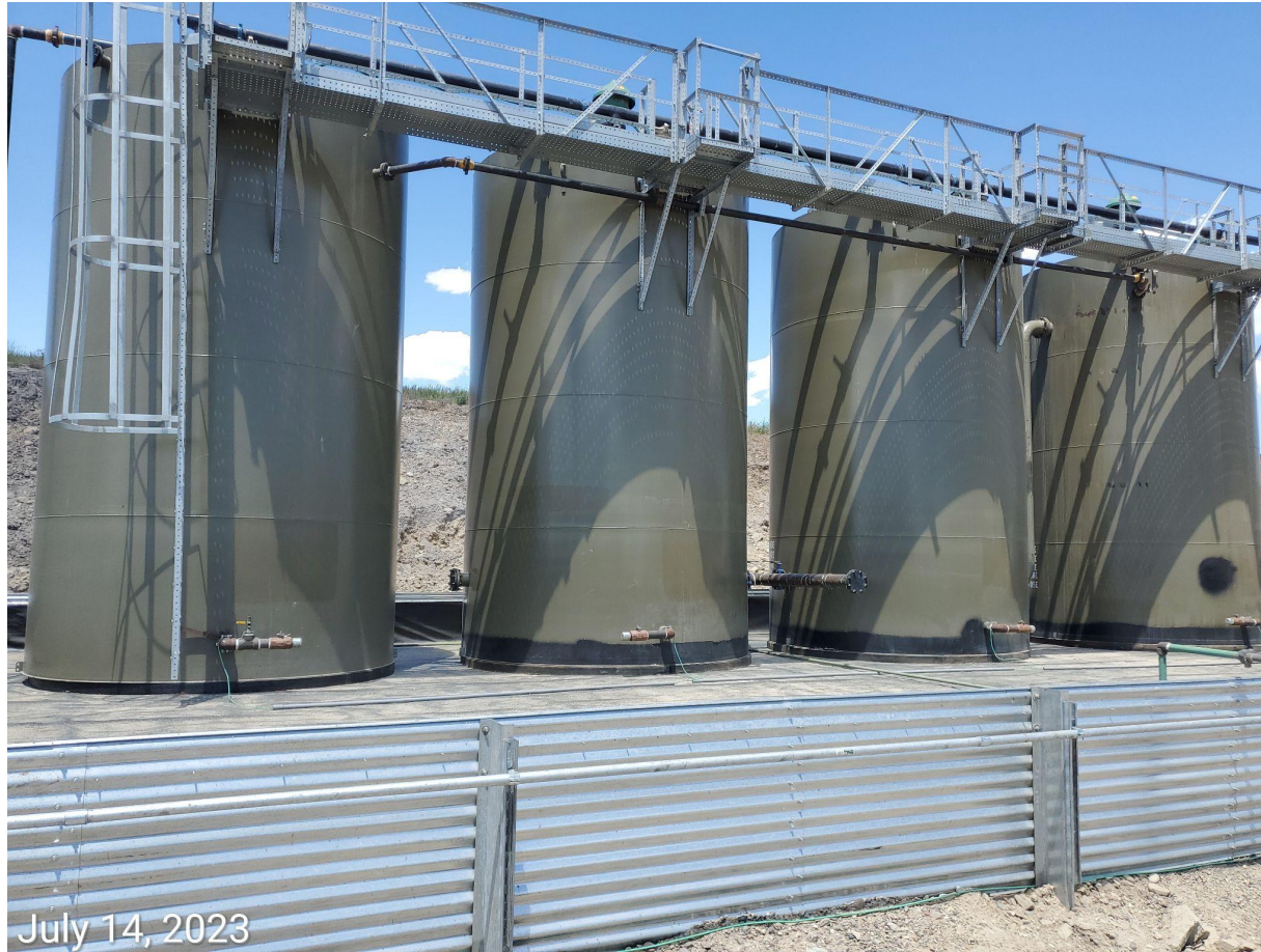
Photo 5: Signage/labels missing from tanks/battery.
