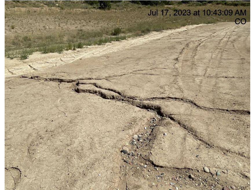
Photo # 3258 Rill erosion (North side of location)
