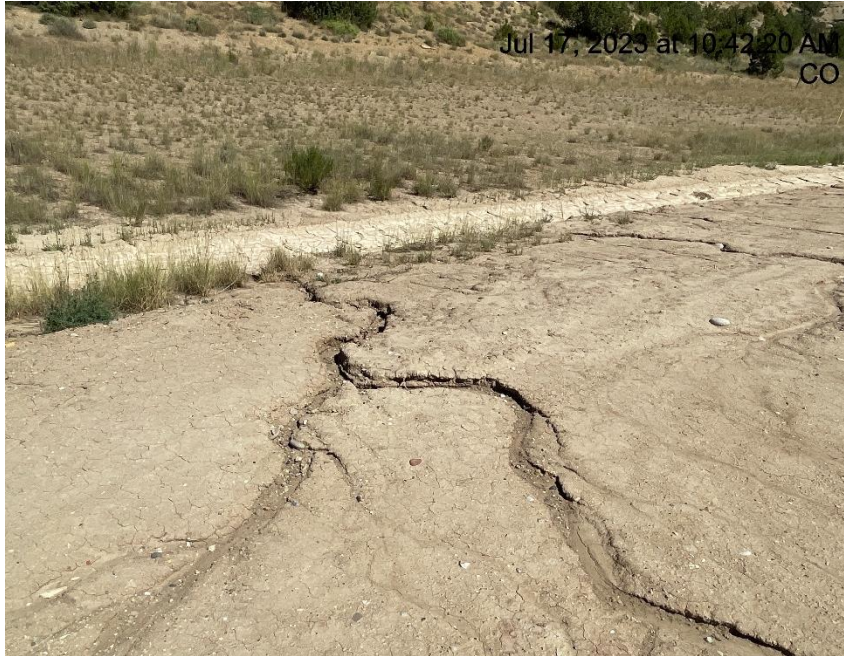
Photo # 3253 Rill erosion (North side of location)
