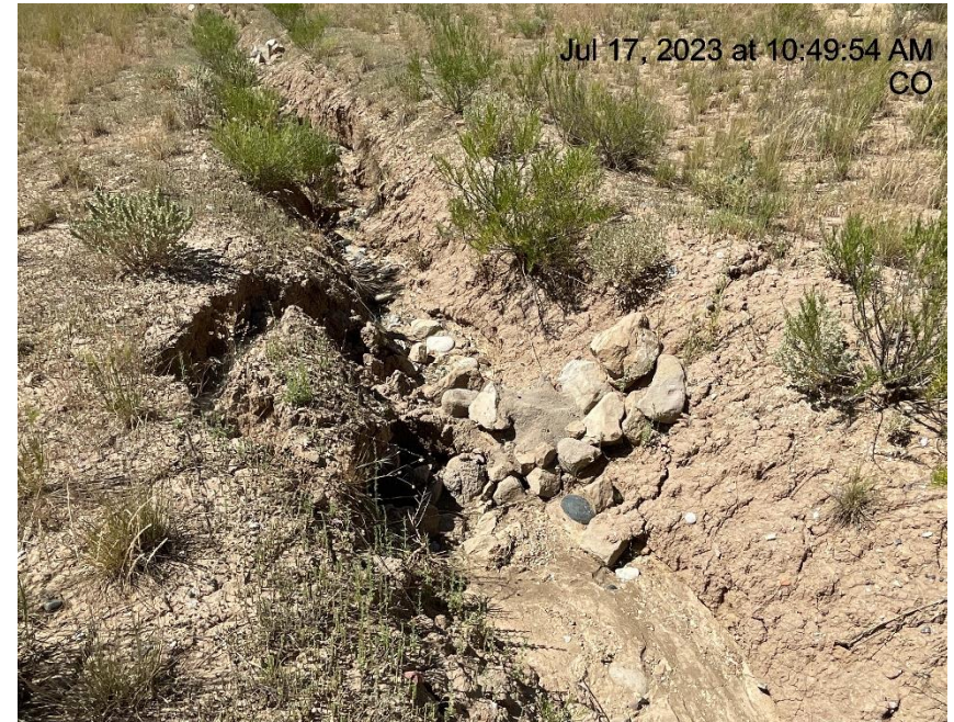
Photo # 3293 BMP's need maintenance/insufficient run on controls
