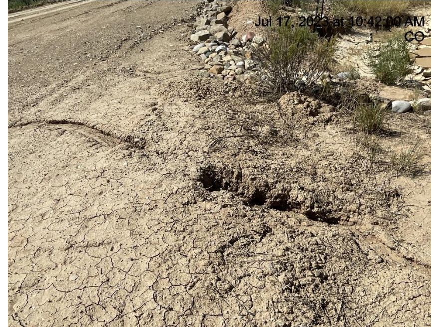
Photo # 3251 Tunnel erosion (N/NW area of pad)
