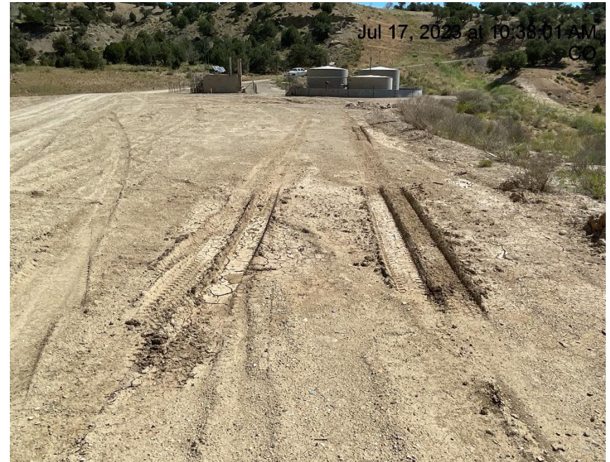
Photo # 3233 Lack of compaction/Stabilization
