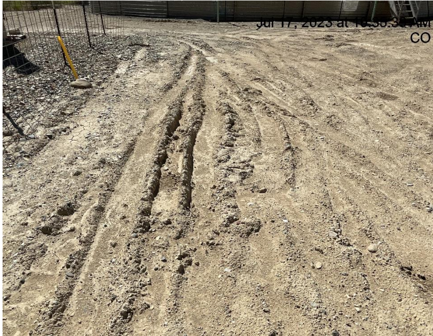
Photo # 3224 Lack of compaction/Stabilization
