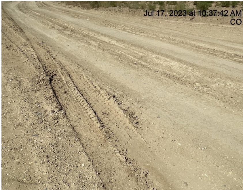
Photo # 3232 Lack of compaction/Stabilization
