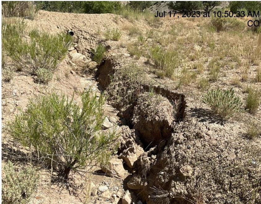
Photo # 3294 BMP's need maintenance/insufficient run on controls
