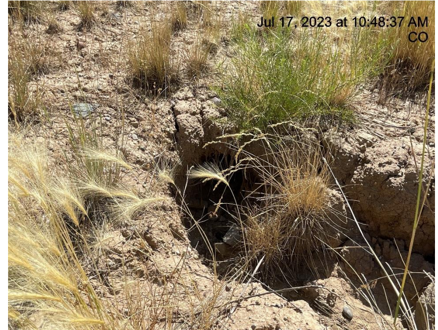
Photo # 3290 Tunnel erosion through berm (N/NE area of location)
