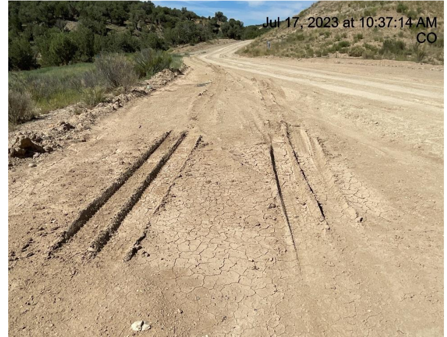
Photo # 3231 Lack of compaction/Stabilization
