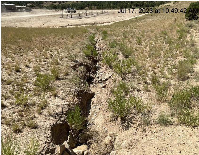
Photo # 3292 BMP's need maintenance/insufficient run on controls
