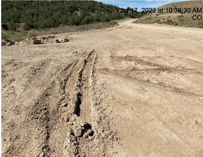
Photo # 3228 Lack of compaction/Stabilization
