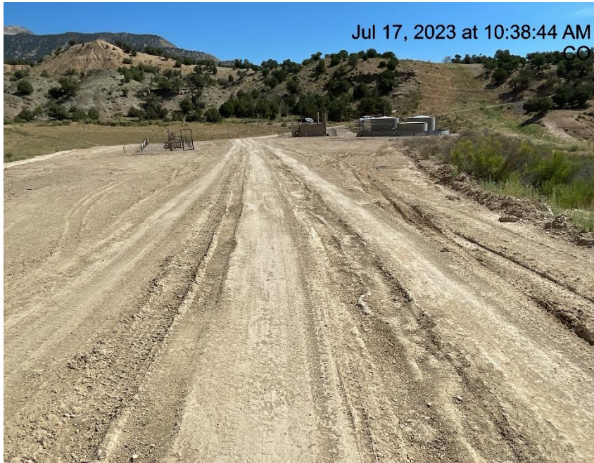
Photo # 3238 Lack of compaction/Stabilization
