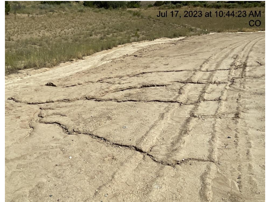
Photo # 3267 Rill erosion (North side of location)
