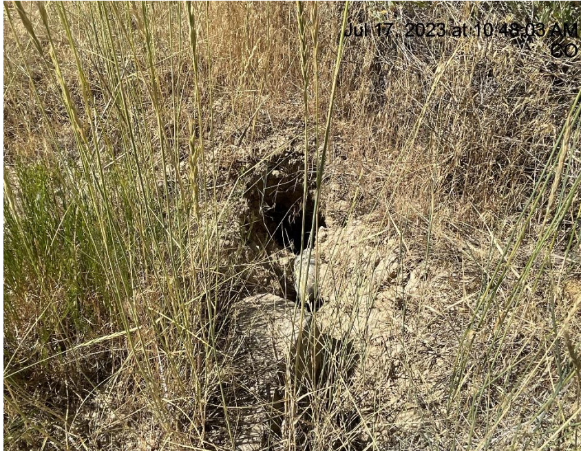
Photo # 3288 Tunnel erosion through berm (N/NE area of location)
