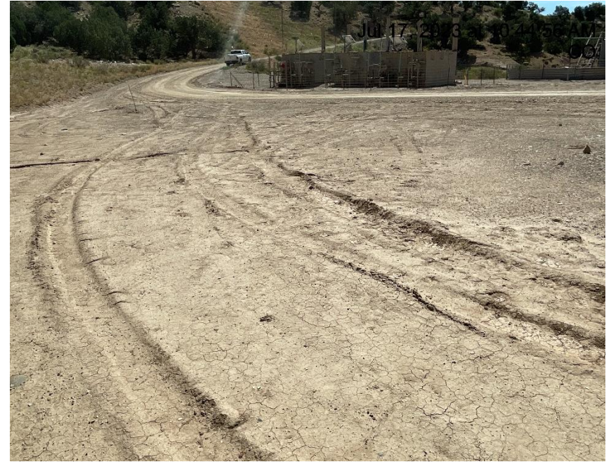
Photo # 3271 Lack of compaction/Stabilization
