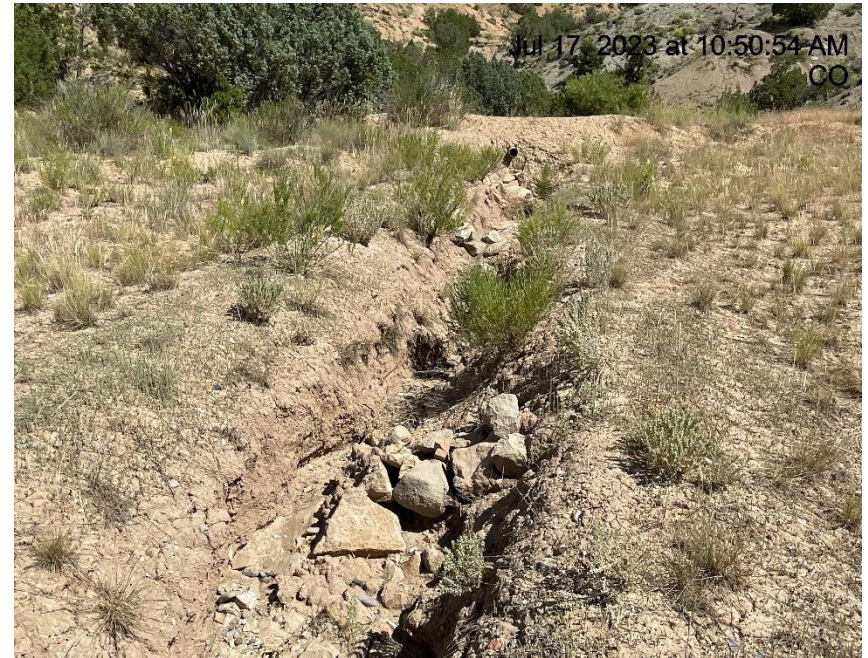
Photo # 3295 BMP's need maintenance/insufficient run on controls
