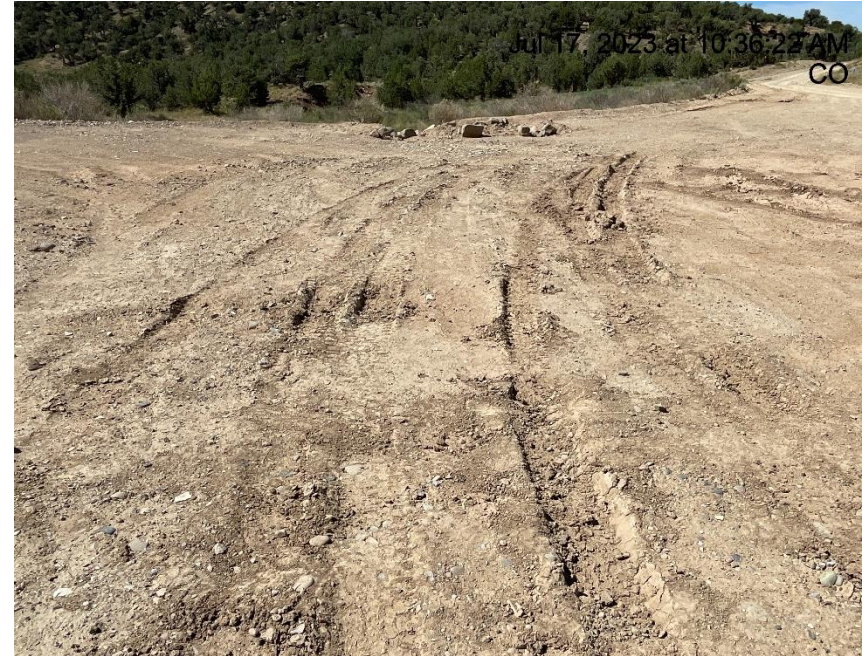
Photo # 3227 Lack of compaction/Stabilization
