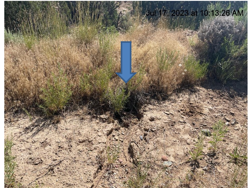
Photo # 3175 Erosion & transport of sediment off location/sediment choking off vegetation/Tunnel erosion going through berm (E/NE area of location)
