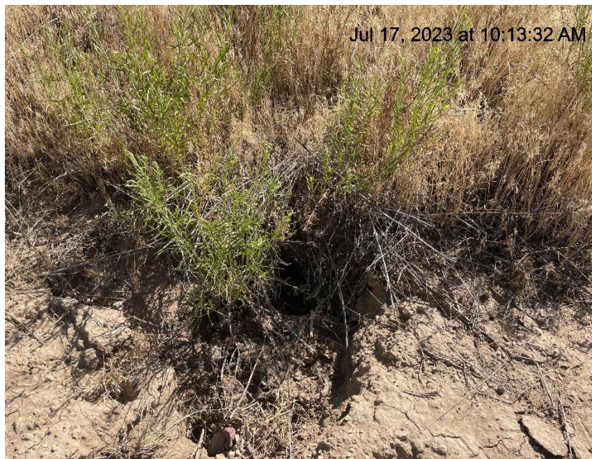
Photo # 3176 Tunnel erosion in berm (E/NE area of location)
