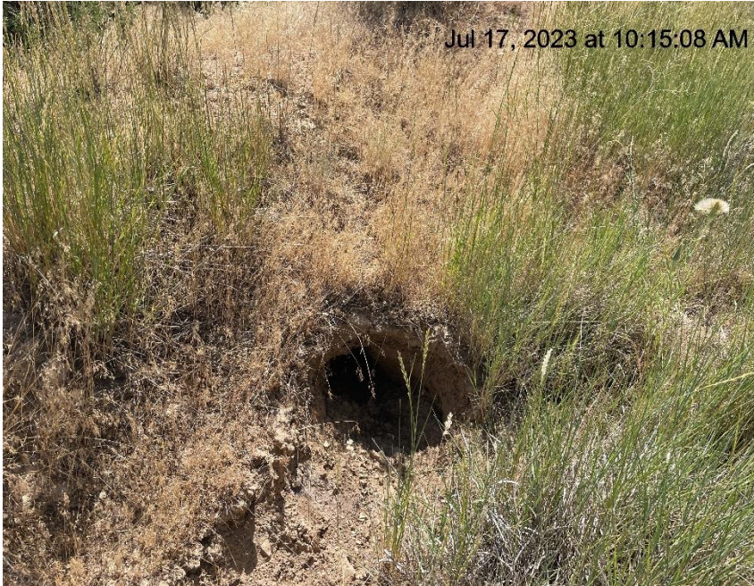
Photo # 3183 Tunnel erosion through berm (E/NE area of location)
