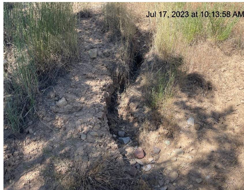
Photo # 3177 Opposite side of berm – tunnel erosion has breached berm & is carrying sediment further offsite & into a drainage (E/NE area of location)
