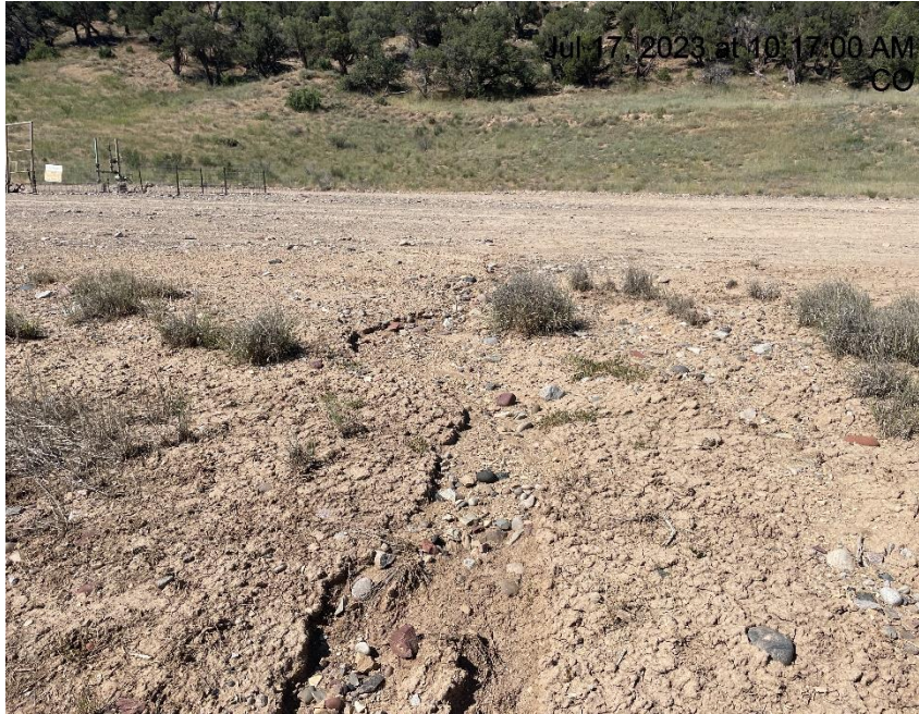
Photo # 3191 Erosion & transport of sediment off location
