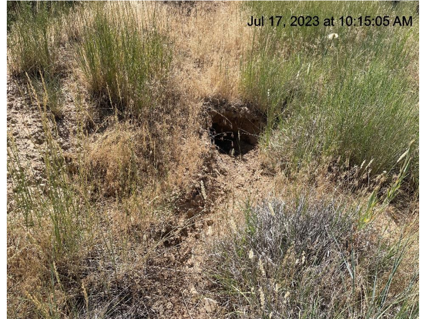
Photo # 3182 Tunnel erosion through another area of the berm (E/NE area of location)
