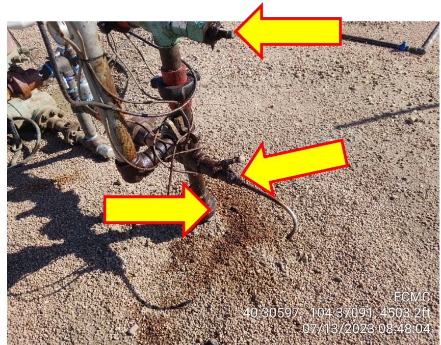
Photo 2 – Stained Soil – Backpressure and Needle Valves appear to be leaking onto ground
