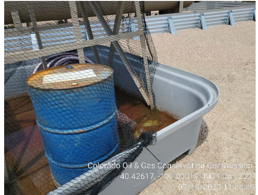
Lube oil tank wildlife protection
