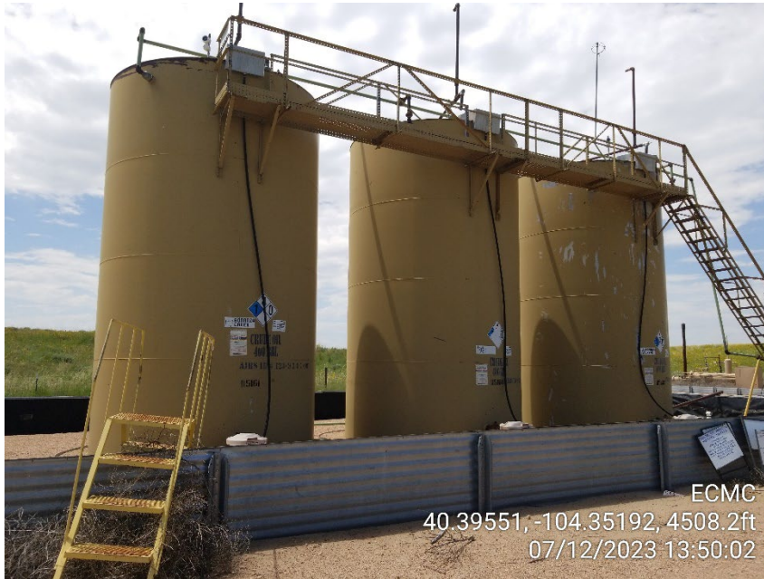
Photo 5 – Tank Battery
