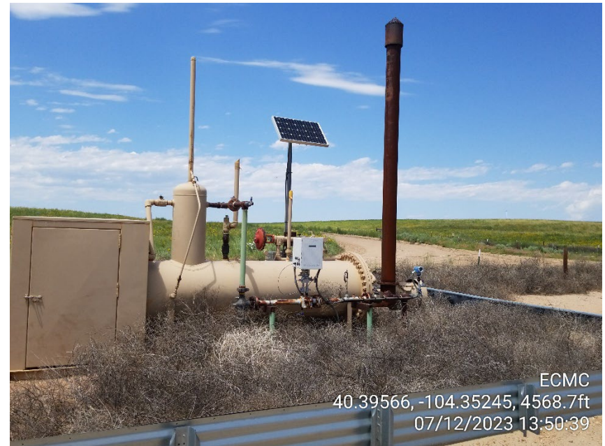
Photo 10 – Separator – Tumbleweed Debris
