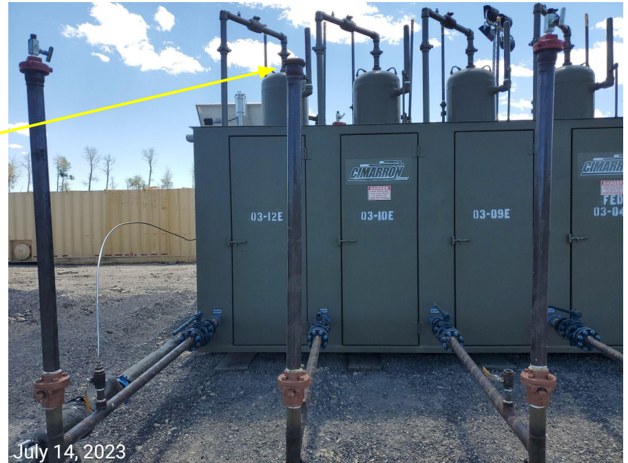
Photo 4: Uncapped/exposed line observed at separator equipment.
