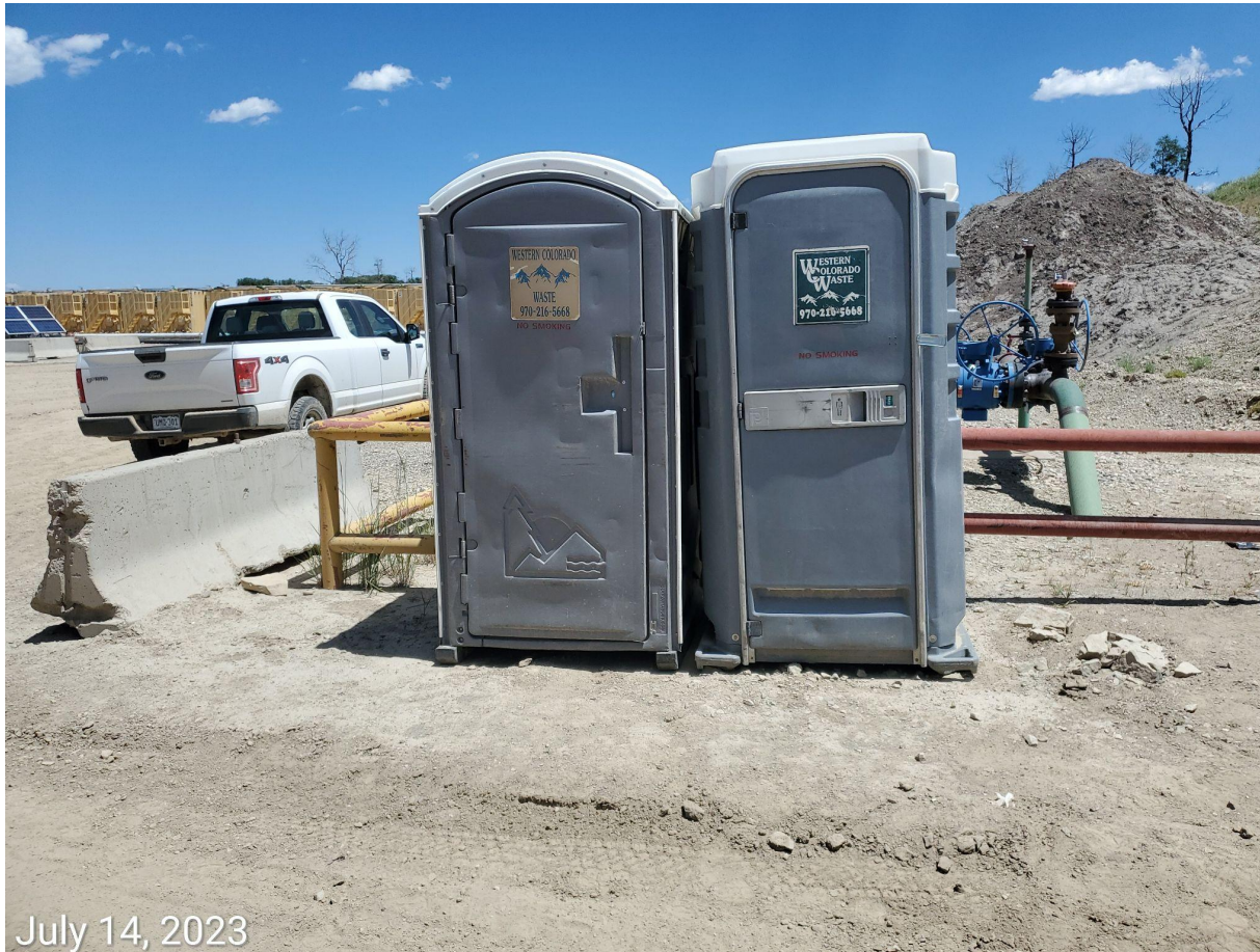
Photo 5: Porta-johns stored at the Location entrance lack required spill prevention/containment BMPs.
