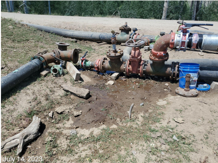
Photo 7: Spill observed at frac lines south of the Location. Fluids observed leaking into the blue bucket containing dark fluids.
