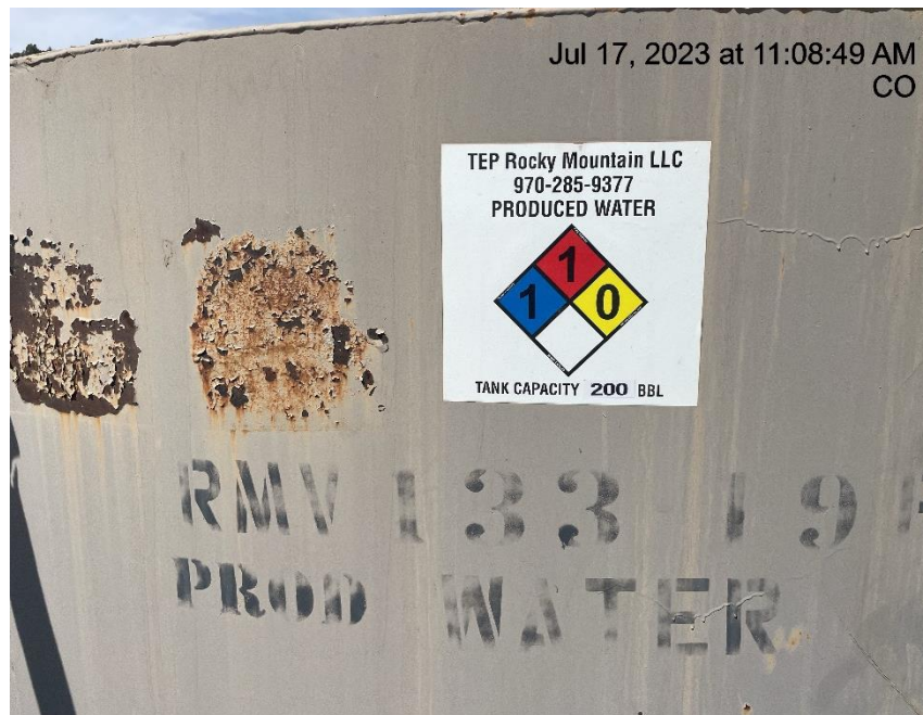
Photo # 3325 Tank label has incorrect capacity
