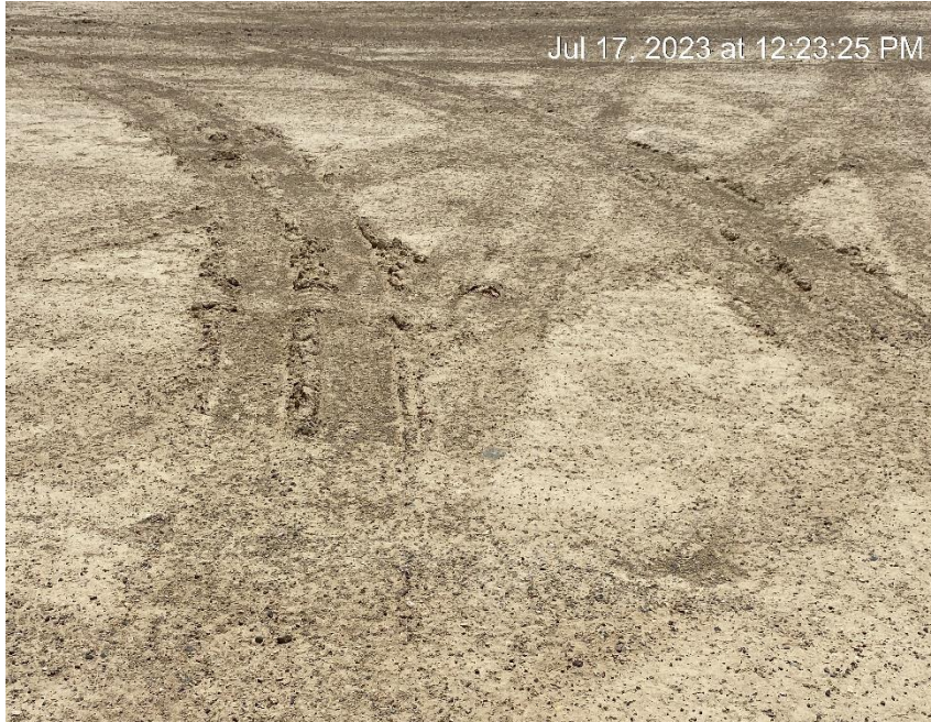
Maintain vehicle tracking BMPs
