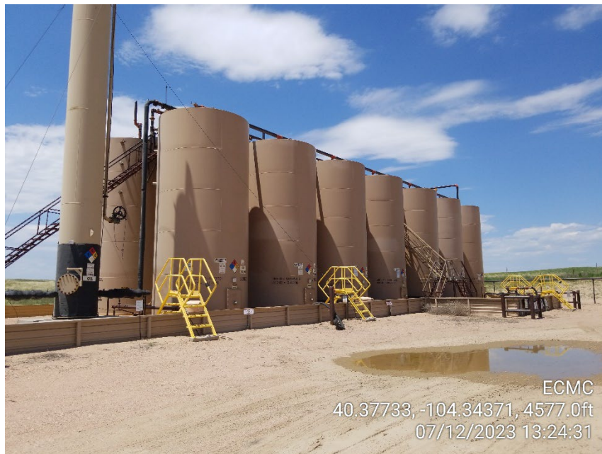
Photo 9 – Tank Battery
