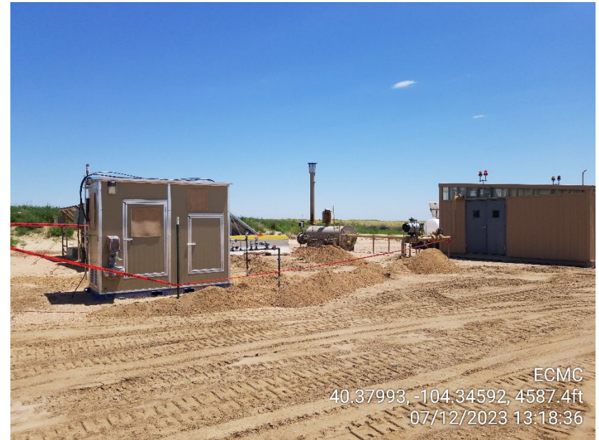
Photo 2 – Instrumental Air Unit and Gas Lift Injection Meter House
