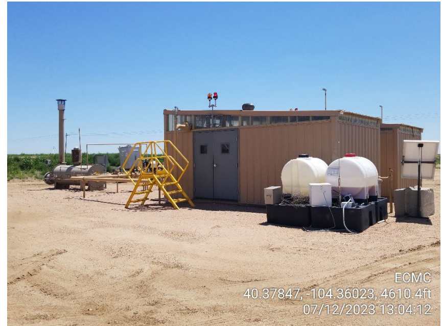
Photo 6 – Gas Lift Injection Meter House
