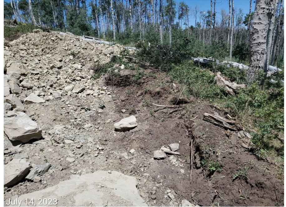
**Photo 9:** Photos taken from the outside perimeter of the stockpile on the east end of the Location. Operator appear to have constructed a ditch utilizing topsoil material. Photos also show stockpile lacks stabilization. Photo right shows material has eroded from the stockpile, filling in the ditch and traveling off-site.
