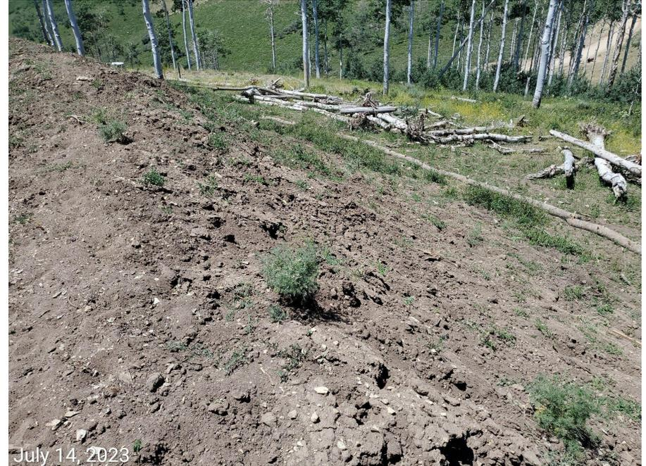
**Photo 3:** Photos 3-4 taken from the topsoil stockpiles on the Location. Photos examples showing BMPs to protect the topsoil from erosion, degradation and weed establishment remain missing or insufficient. Soils predominantly bare and at risk to erosion. Vegetation observed on topsoil stockpiles Undesirable Plant Species such as amaranth, various introduced mustard species, prostrate knotweed, etc...
