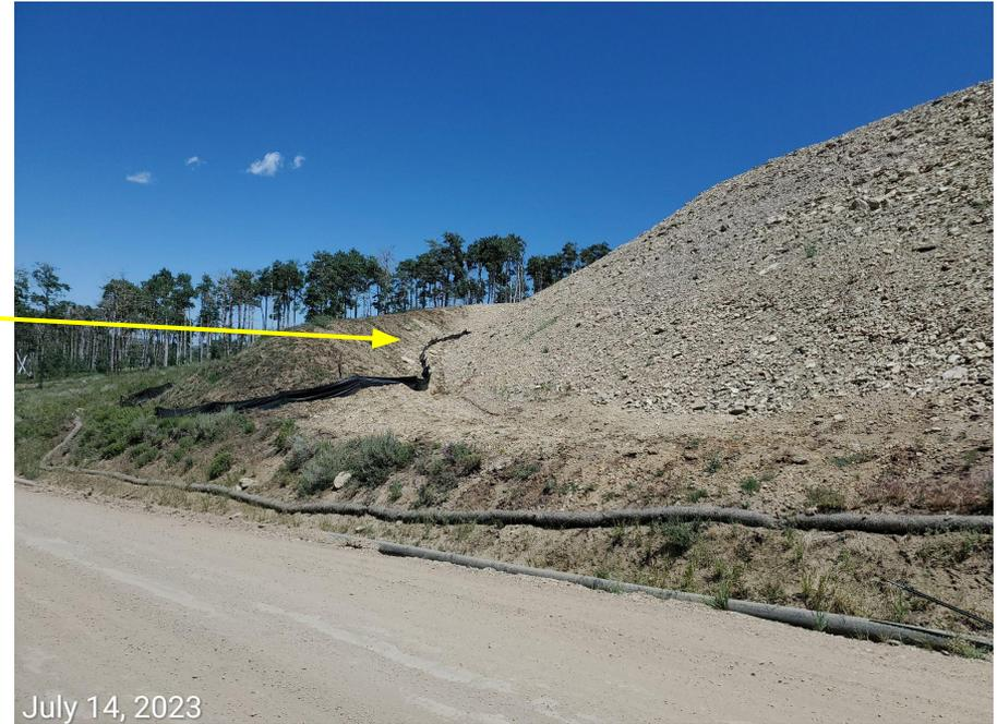
**Photo 14:** Photo left shows the topsoil stockpile on the northwest end of the Location as observed during the 10/17/2022 inspection. Photo right shows large areas of the topsoil stockpile have been covered by fill/subsoil material.
