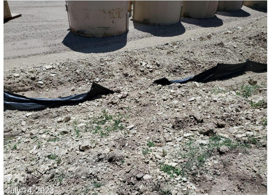
**Photo 5:** Photos 5-6 examples showing silt fence installed on the Location have not been maintained in proper functioning condition. Photos also show BMPs to ensure topsoil remains segregated from the fille slope/subsoils are inadequate on the Location.
