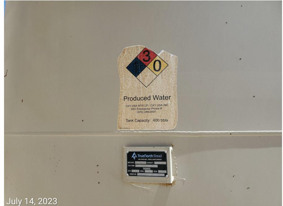
**Photo 16:** Photo shows tanks stored on the north end of the Location. Photo right an example showing labels on the tank are missing, or not per 605.h requirements.
