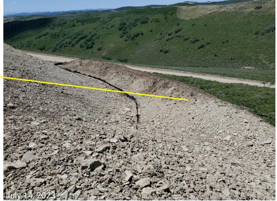
**Photo 13:** Photo left shows the topsoil stockpile on the northwest end of the Location as observed during the 10/17/2022 inspection. Photo right shows that the majority of the topsoil stockpile has been buried beneath fill/subsoil material; areas of the topsoil stockpile below arrow in the right photo (foreground of photo left) have been completely covered.
