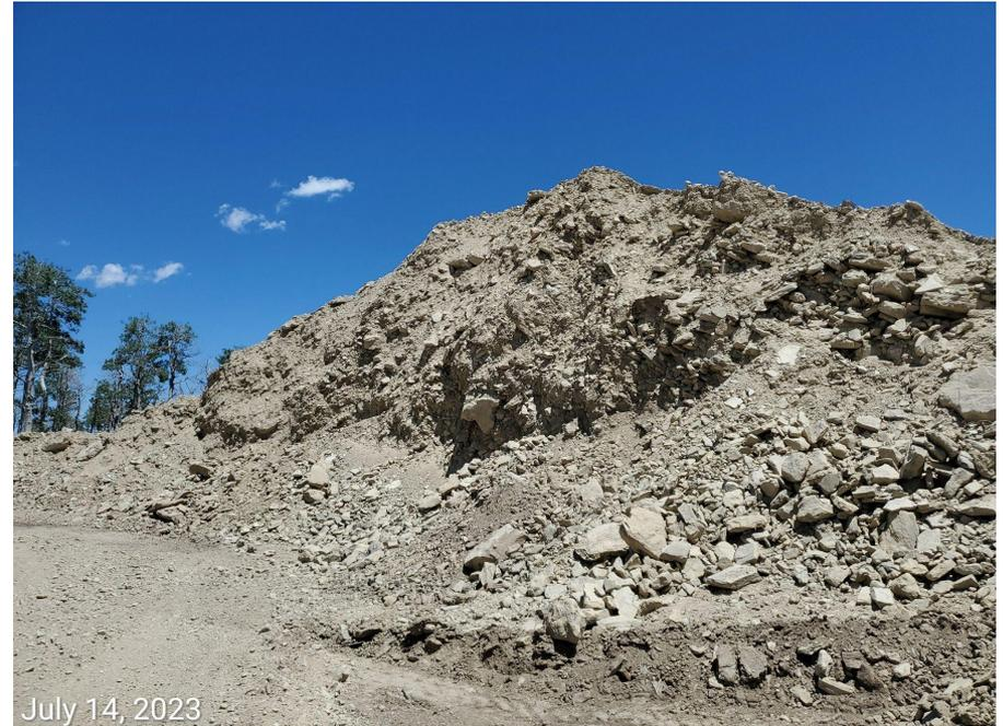
**Photo 7:** Photos 7-8 taken from the northeast corner of the pad. Photo shows unstabilized soil stockpile. Stockpile lacks stabilization, or adequate BMPs to minimize erosion/degradation. Potential safety issues also exist due to the unstabilized steep slopes above the pad.
