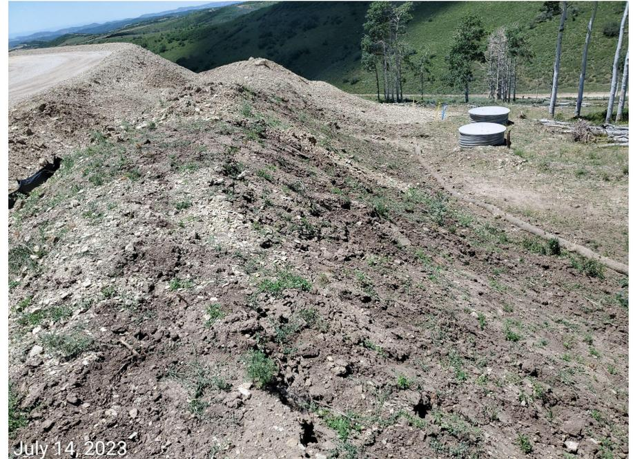
**Photo 12:** Photos 12-15 taken from the topsoil stockpiles on the Location. Photos examples showing Operator placed subsoils/fill material on top of the topsoil stockpiles on the Location.
