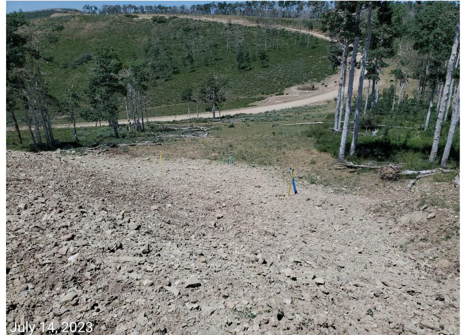
**Photo 11:** Photos taken from the north end of the Location. Photos show perimeter stormwater BMPs to minimize erosion, degradation and sediment transport remain missing or insufficient.
