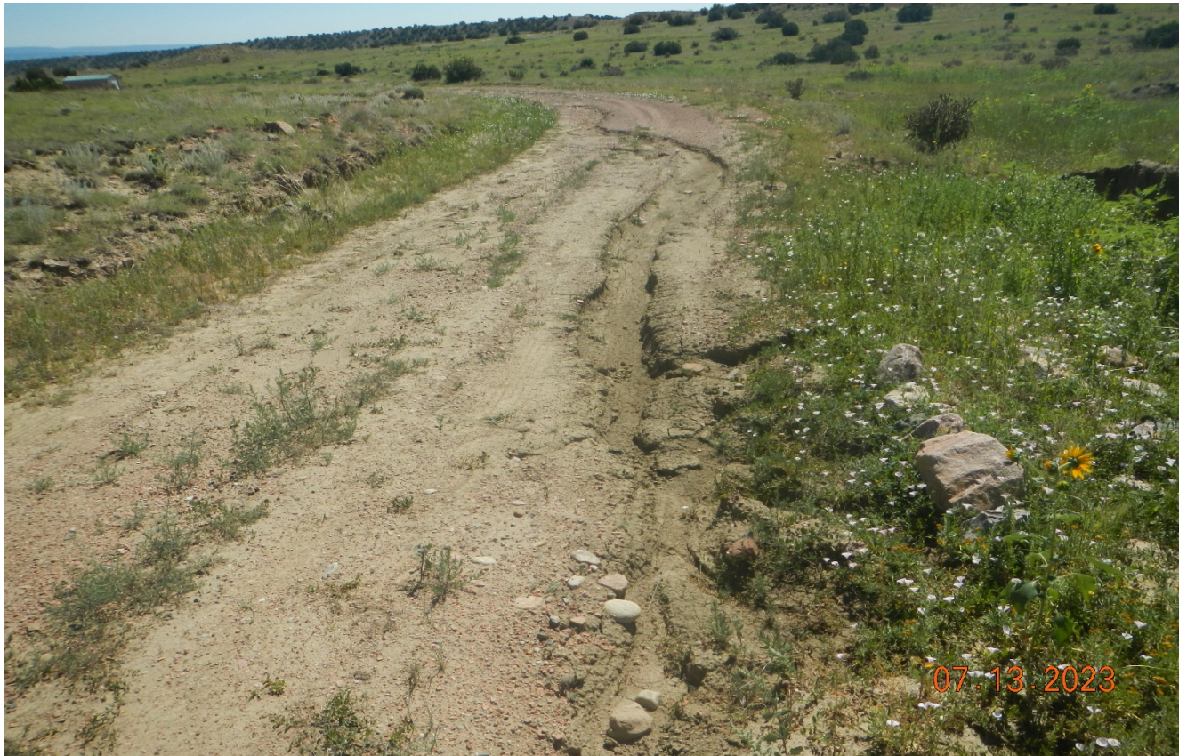
Photo 1. Facing northeast along the access road. There is erosion occurring along the road that needs to be repaired.
