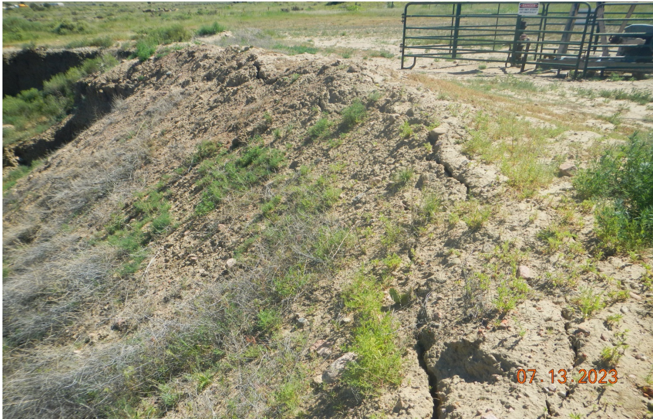
Photo 6. It appears additional soil was brought into the erosion gully near the well however, this area is not stabilized. There are cracks along this area which indicate soil movement which needs to be stabilized.
