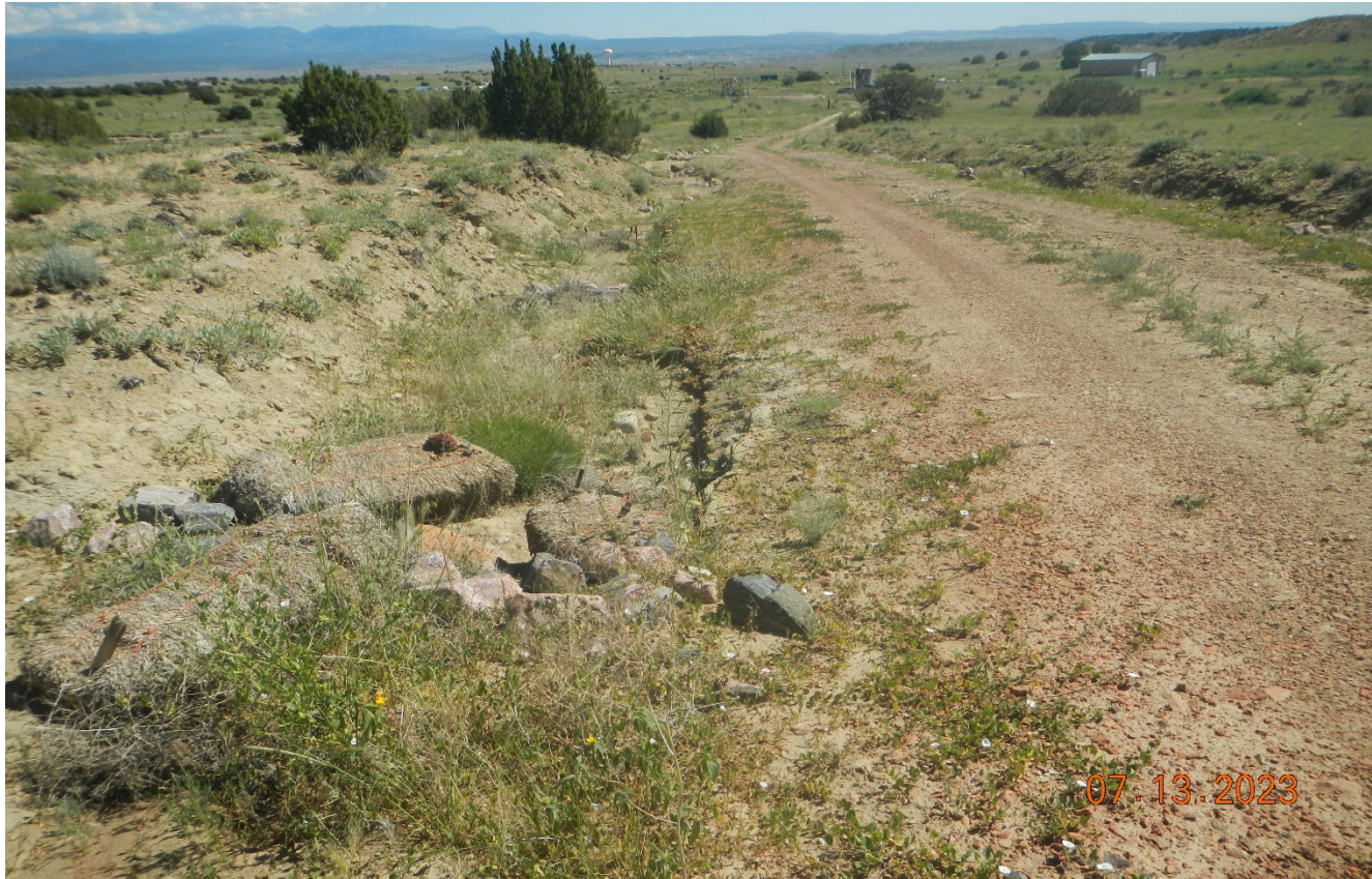
Photo 2. Facing northeast along the access road. BMP's along the road side are not maintained and have filled in with sediment.
