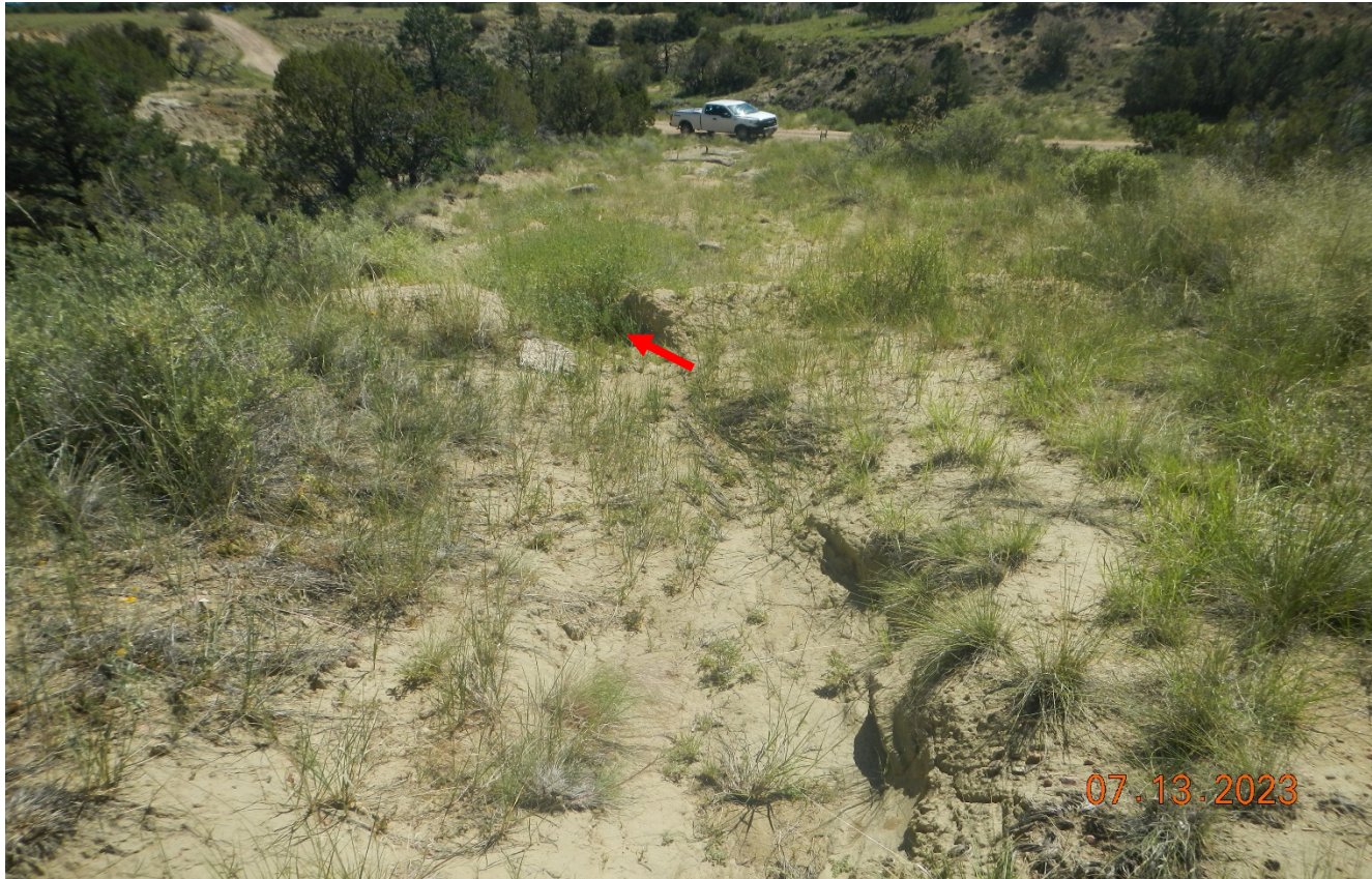
Photo 4. Further up along the access road facing northeast. There is an erosion channel directed down to the left side shown at red arrow.
