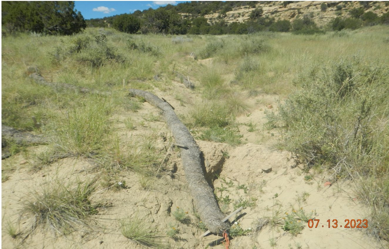
Photo 6. Facing southwest along the former access road. It appears that the stormwater from the location is directed down the road which is causing erosion issues shown in previous photos. Wattles that were installed have been washed out.
