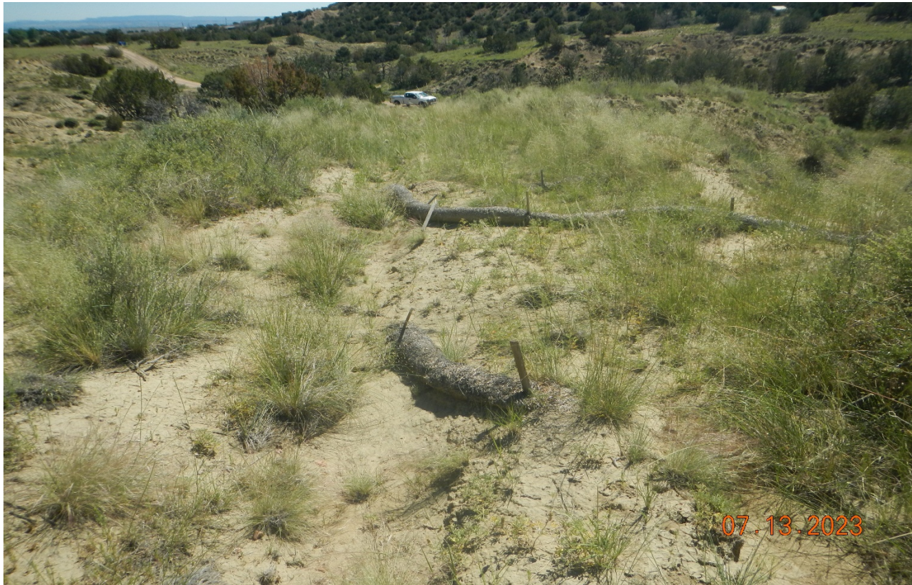
Photo 7. Facing back northeast along the former access road. It appears that the stormwater from the location is directed down the road which is causing erosion issues shown in previous photos. Wattles that were installed have been washed out.
