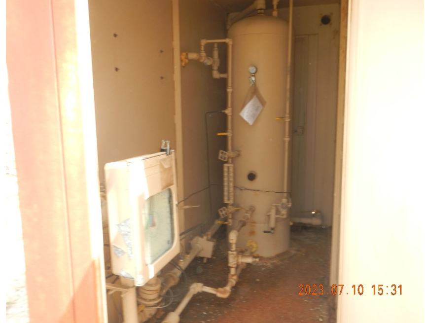
4. View of Gas Meter Run and Vertical Separator inside shed.
