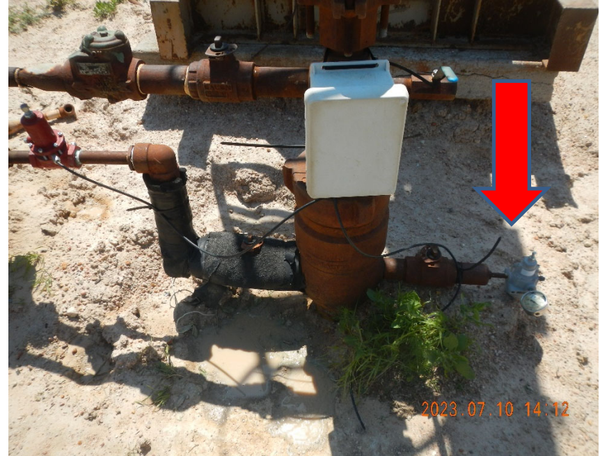
8. Wider view of Wellhead and venting Regulator on right side of frame under red arrow.
