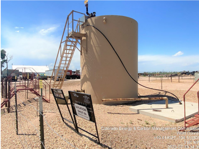
Photo #3 Trebor B 11-22 Battery site Inactive | Shut-down Tank(s): SE corner
